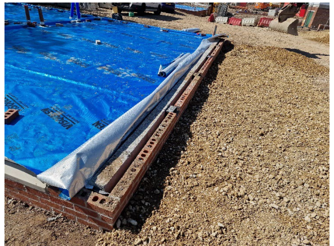
Figure 2 – Sufficient vents.
