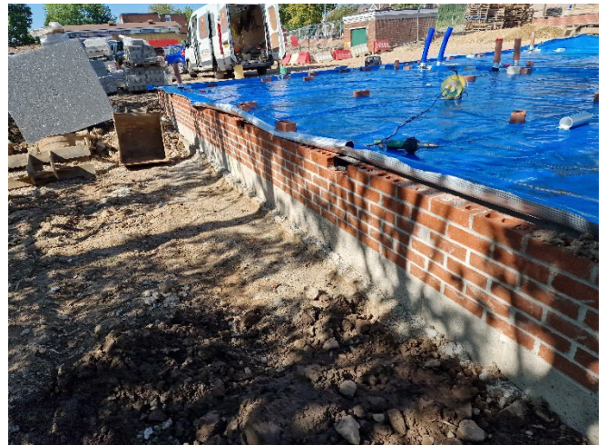
Figure 4 – Sufficient vents.
