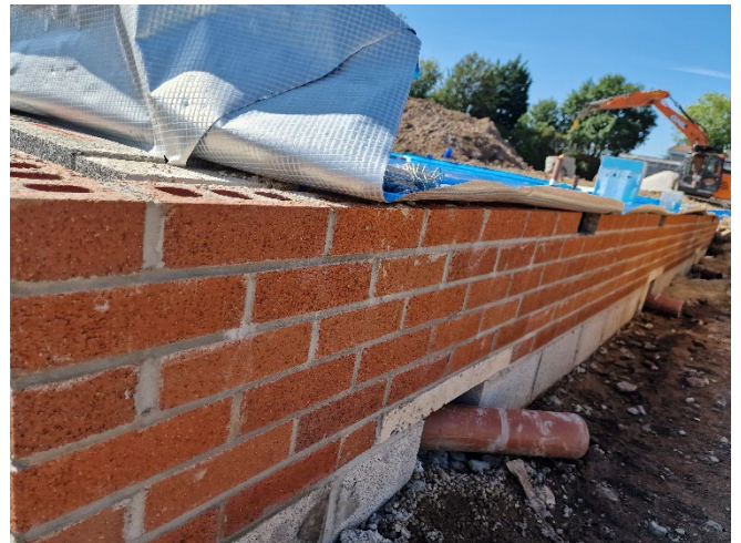
Figure 4 – Sufficient vents.
