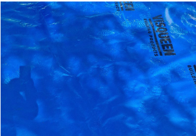
Figure 5 – Hand Welded Seams
