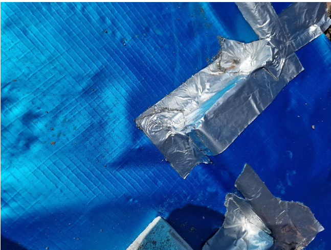
Figure 3 – Corners installed using detailing tape giving sufficient coverage of cavities
