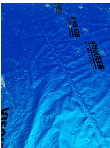
Figure 5 – Hand Welded Seams
