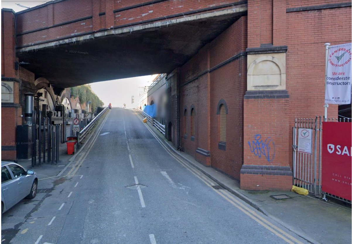
Access under low bridge on Trafford Street
