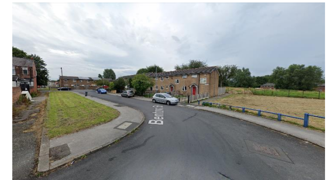
View of two storey terraces adjacent to the sites east boundary, along Benton Street. Showing right of access path next to existing end terrace.
