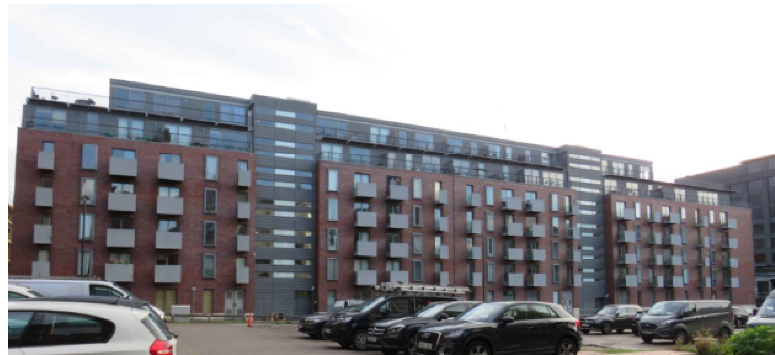
PICTURE 04 - BREWER STREET ELEVATION - SHOWING BOTH STAIRWELLS
