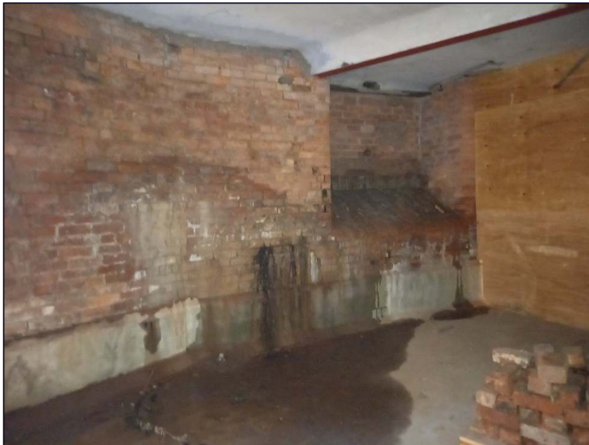
Plate 24: Southern end of the south-east elevation of Area 1 showing the angled wall and blocked window, lower ground floor
