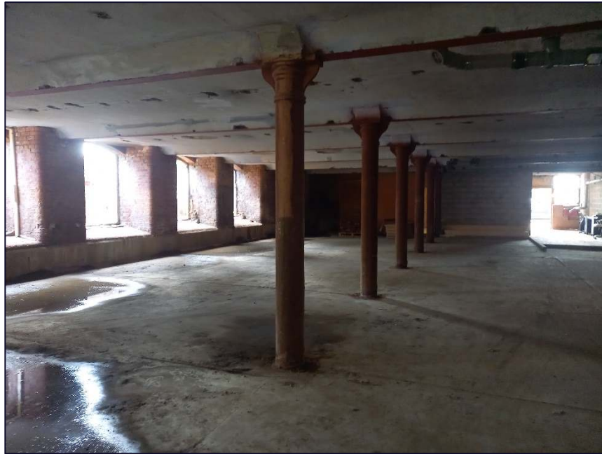
Plate 19: View looking south-west showing Area 1 with concrete floor, metal columns and concrete ceiling
