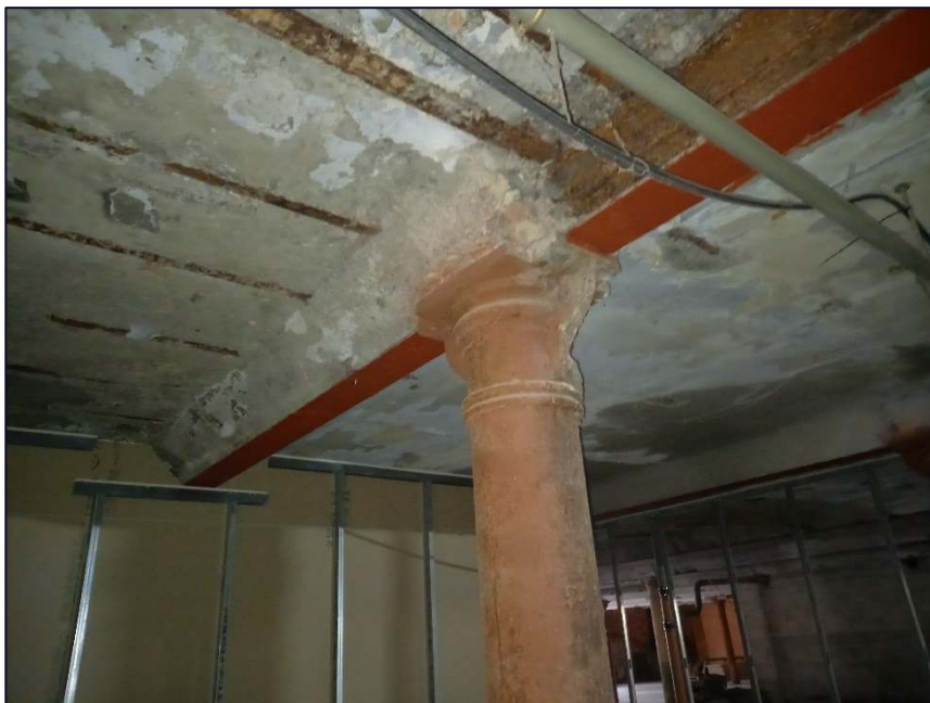
Plate 26: Detail of one of the columns in Area 4
