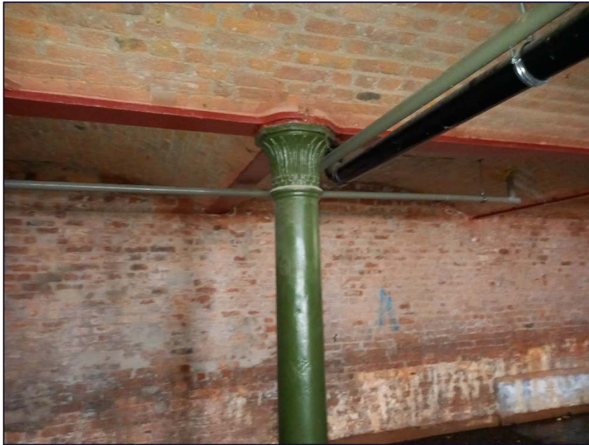
Plate 31: Detail of one of the cast iron columns with decorative capital, Area 3
