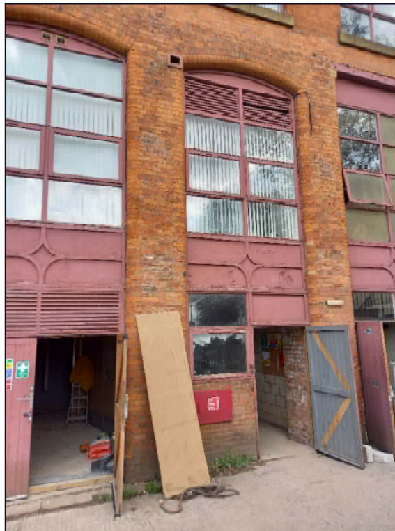
Plate 11: Detail of some of the two-storey door/window combinations in the south-west elevation of "B" mill
