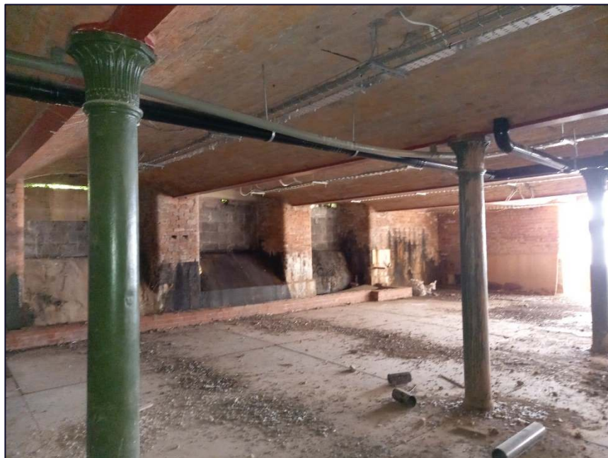
Plate 30: View looking south-east in Area 3 showing the concrete floor, decorative columns and brick jack arches, lower ground floor
