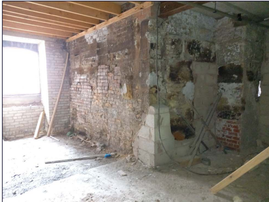
Plate 29: View looking south showing the rectangular feature within Area 2 that has been modified and now includes stonework, brick and concrete blocks
