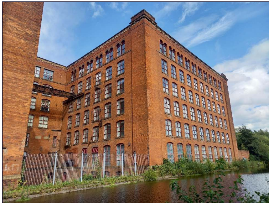
Plate 7: View looking north from the south side of the Rochdale Canal showing the north-eastern block ("A" mill), with the lower ground floor shown to be lower than the canal as can be seen in the courtyard between the two blocks
