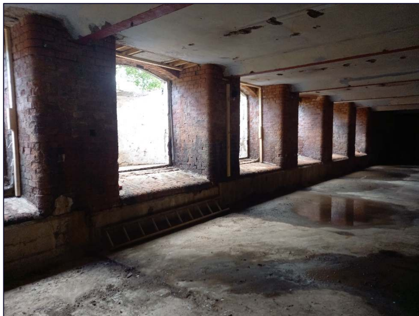
Plate 22: View looking east towards the canal showing the south-east elevation of Area 1
