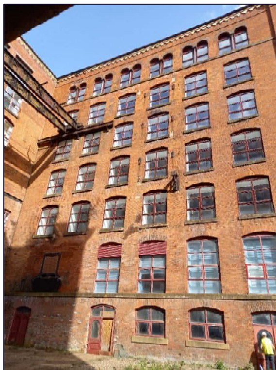
Plate 18: South-east facing elevation of Mill "A" which faces into the courtyard
