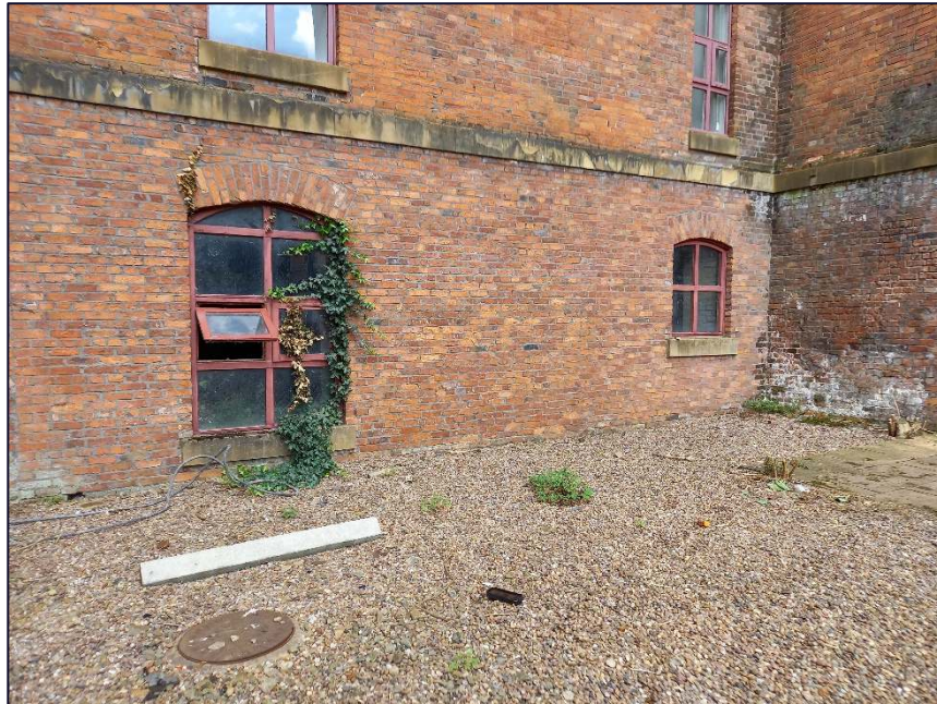
Plate 17: Detail of the two windows in the lower ground floor of the south-east elevation of Area 2
