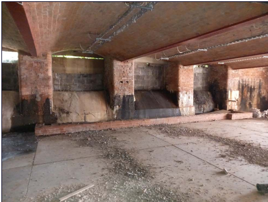
Plate 34: Blocked window openings, south-east wall of Area 3
