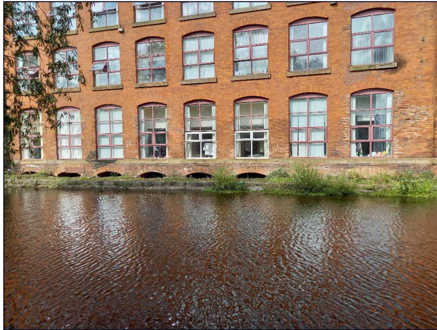
Plate 9: South-east elevation of the south-western block showing the recently cleared out openings which light the lower ground floor
