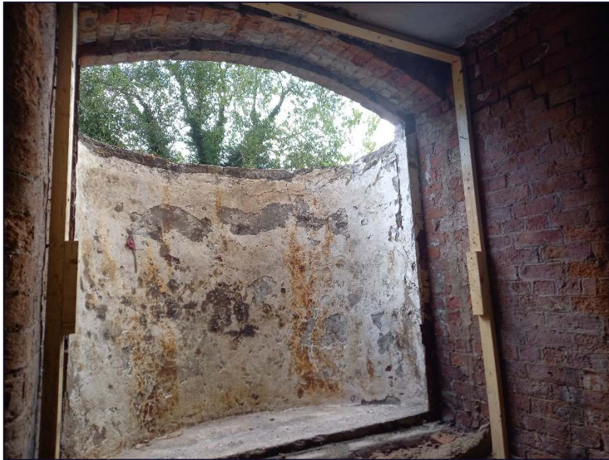
Plate 23: Detail of one of the lower ground floor windows with semi-circular recess. These are set below the top of the side of the Rochdale Canal
