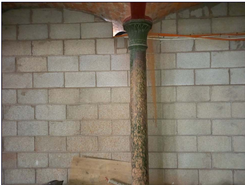
Plate 32: View looking north-west showing one of the columns and a concrete block internal wall in Area 3
