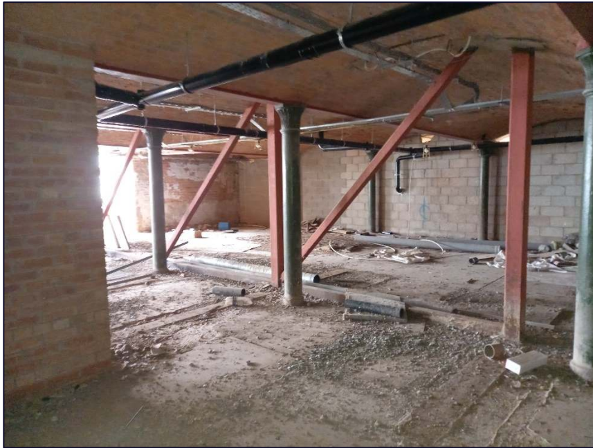
Plate 33: View looking north-west showing Area 3
