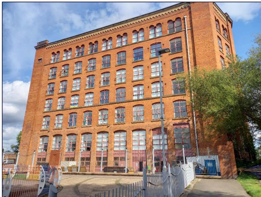
Plate 10: South-west elevation of the south-western block which faces onto the children's playground
