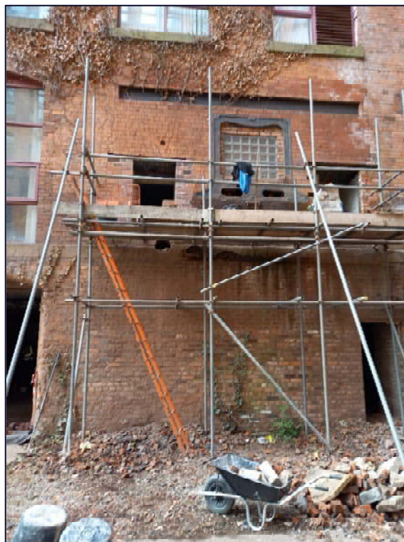
Plate 14: Northern end of the north-east elevation of “B” mill showing the transmission window on the ground floor (above the lower ground floor)
