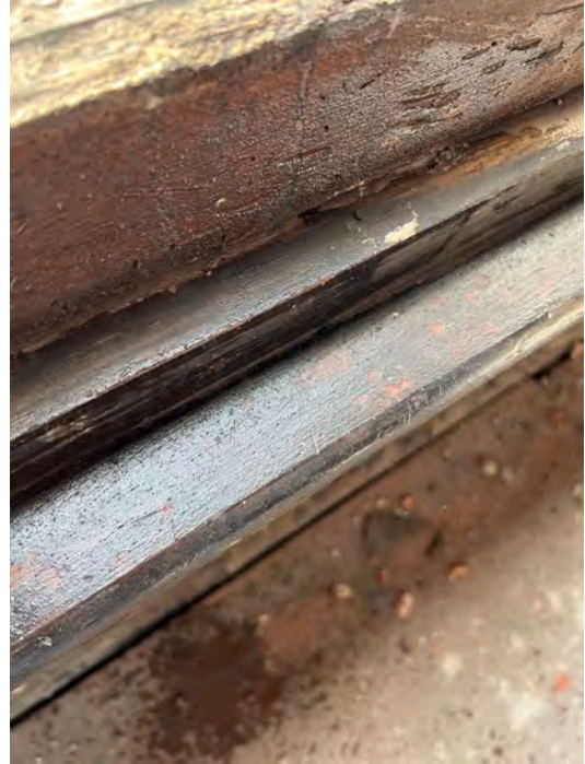
Fig.10 Cill shows single layer of black paint on timber.
