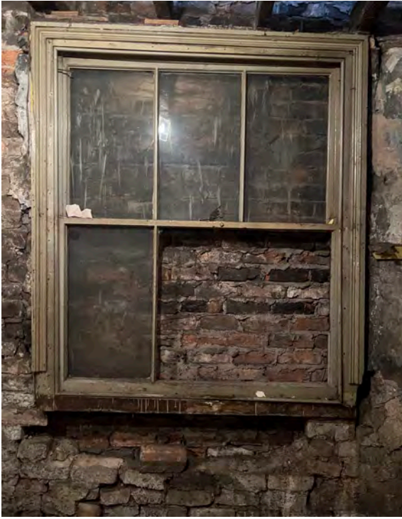
Fig. 12 First floor rear window that has been bricked up.
