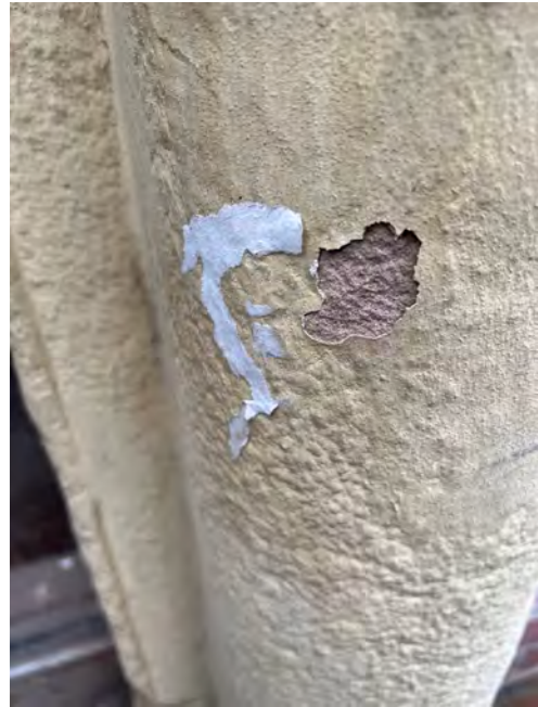
Fig. 23 Removal of single layer of paint revealed original masonry beneath
