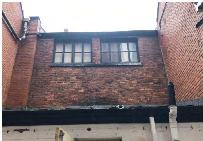
Fig. 4 Rear elevation windows and lintels.
