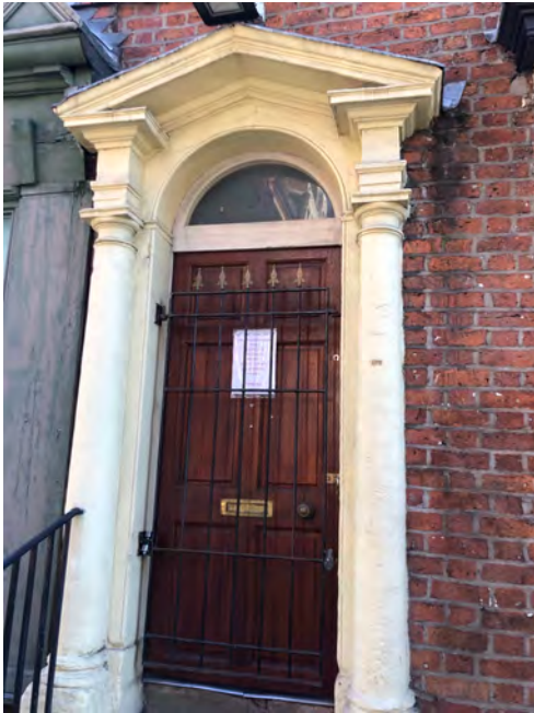
Fig. 22 Columns and portico to entrance.
