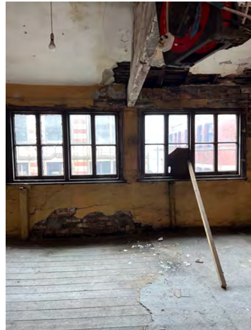
Fig 2. Internal windows to front of building.
