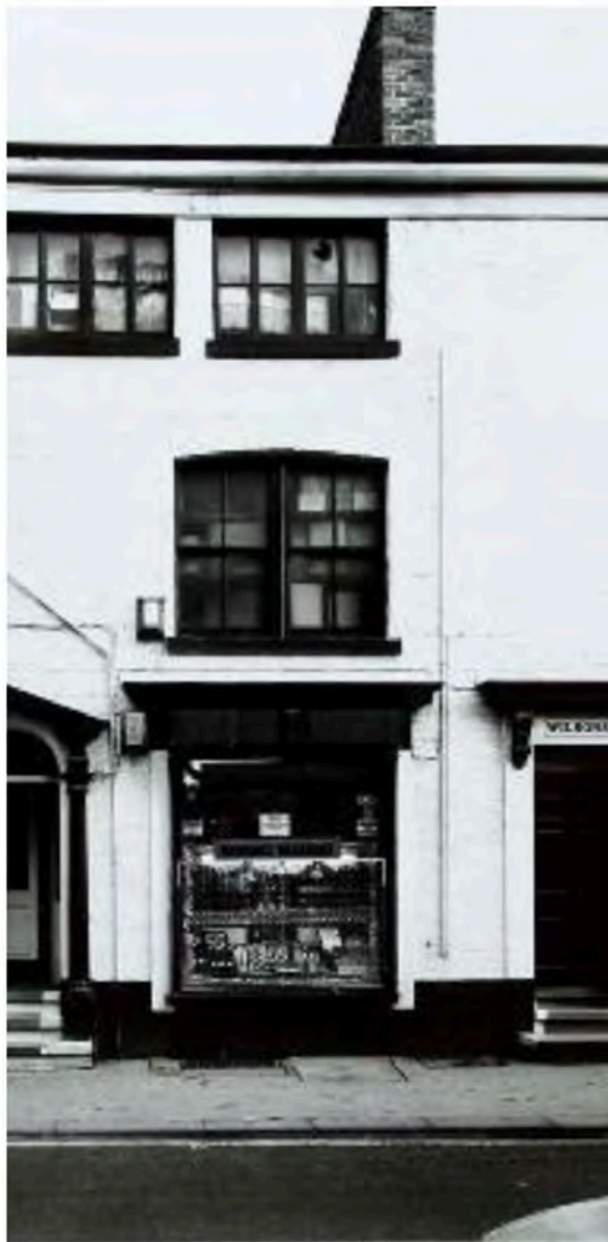
Fig. 26 Photo from Heritage Statement showing all cills, window frames and columns painted black.
