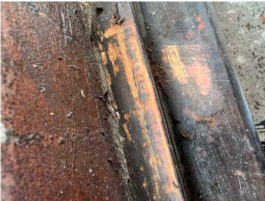
Fig.10 Cill shows single layer of black paint on timber.
