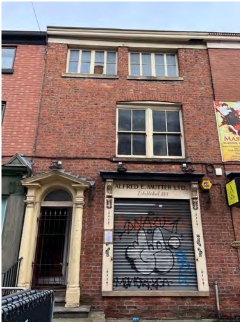
Fig.1 Front Elevation windows and masonry
