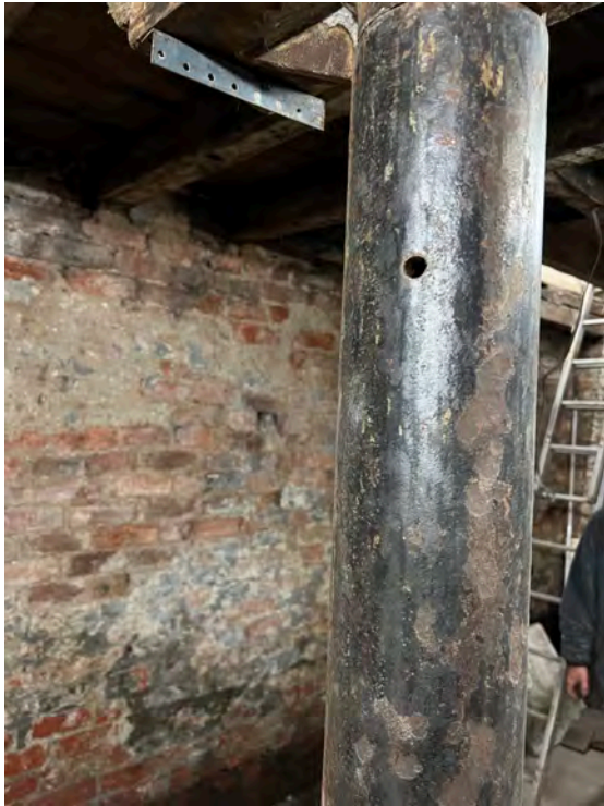
Fig. 16 Column 1 the largest in diameter.
