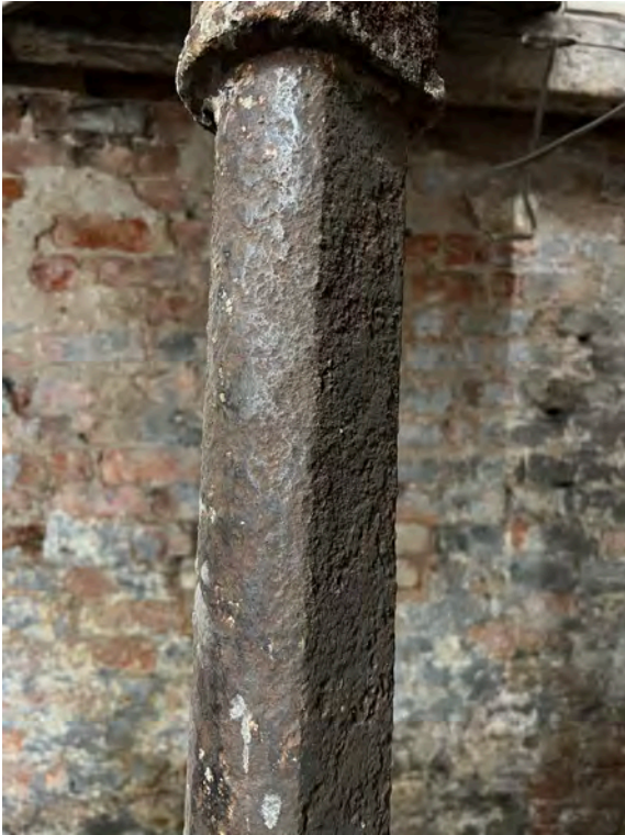
Fig. 20 Column 3 has a flat edge.
