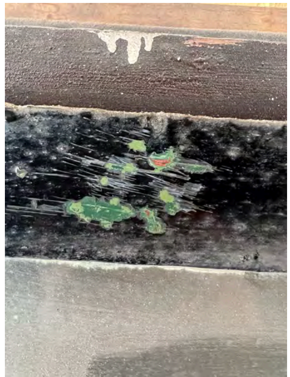
Fig. 8 External side of second floor window removal of top layer reveals a bottle green paint colour below and timber beyond.
