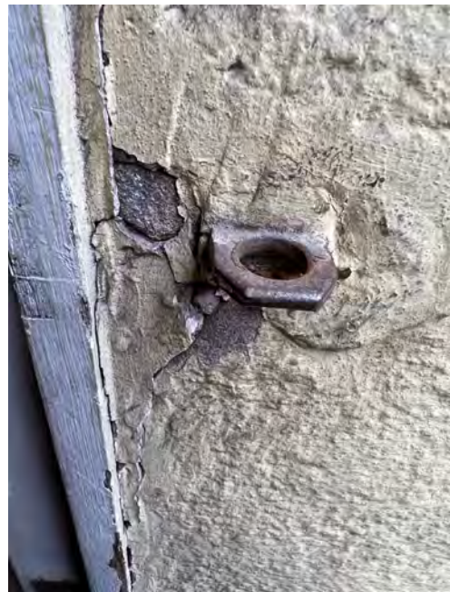
Fig.25 Loose paint shows stone beneath
