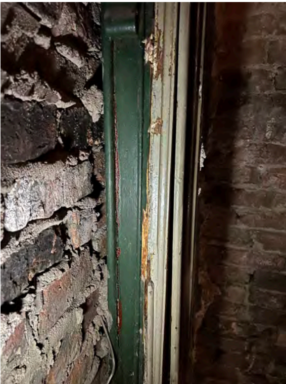
Fig. 14 Showing the bottle green paint that would have been on the exterior of the window before it was bricked up.
