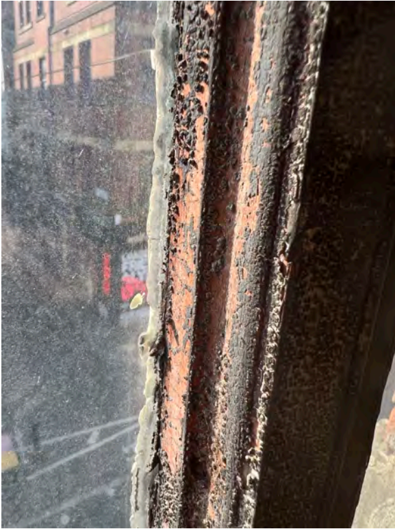
Fig. 5 Internal second floor front window. Single layer of black paint on existing timber frame.
