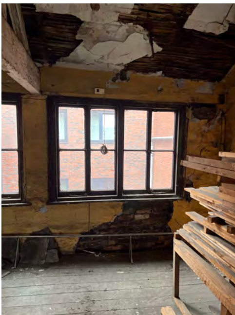
Fig. 3 Internal windows to rear.
