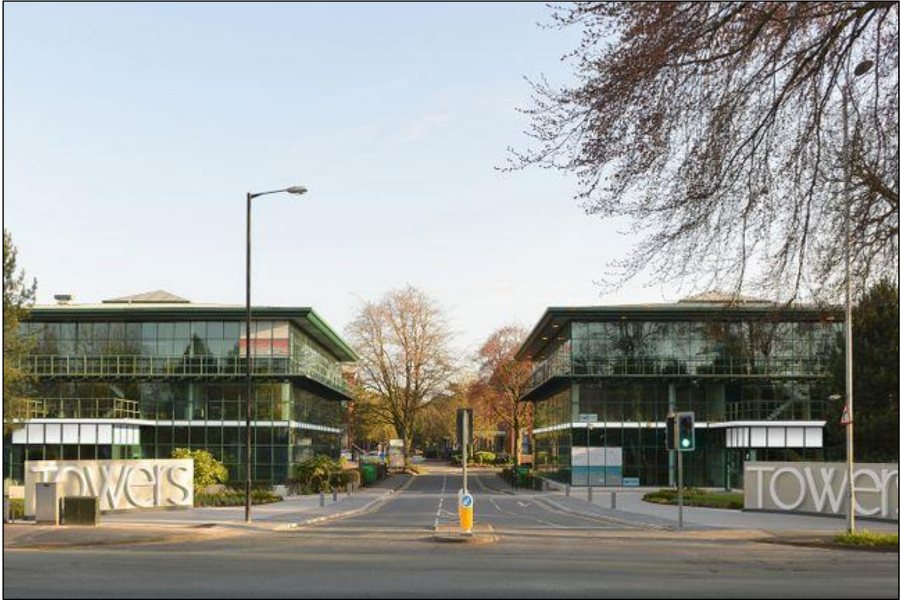
Figure 1. Entrance from Wilmslow Road
