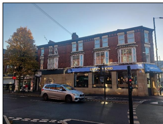
Figure 5: View of 571 - 575 Wilbraham Road frontage.
