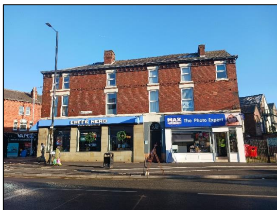
Figure 4: View of adjacent properties (436 Barlow Moor Road (right) and 575 Wilbraham Road (left)).
