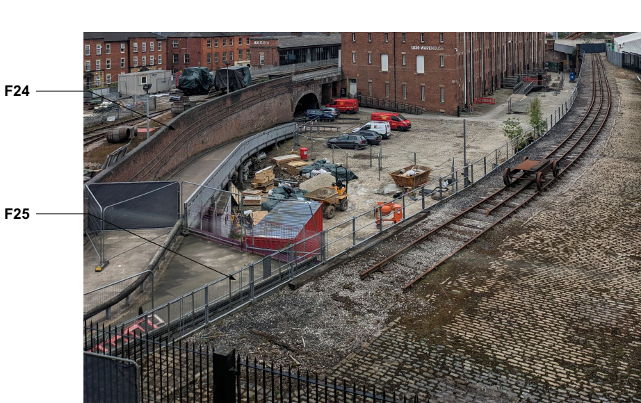
F25 - Existing Balustrade retained
