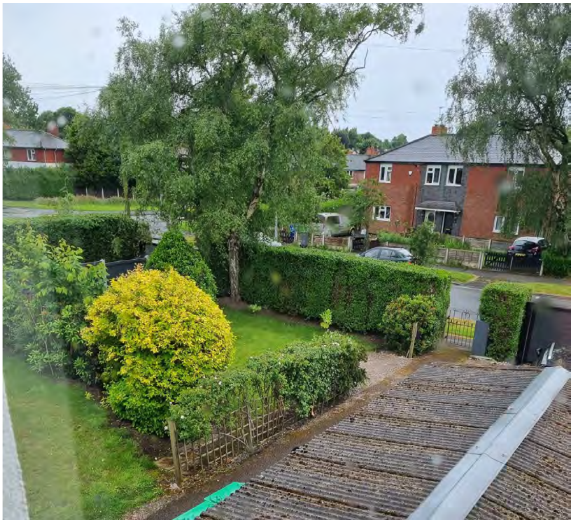
View of the roof of the garage showing assumed asbestos roof sheeting
