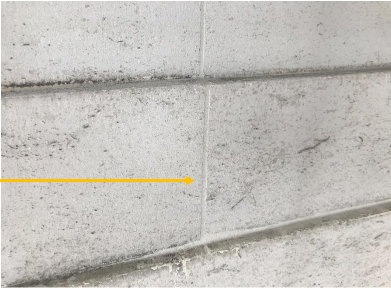
Widened masonry joints forming a chase. Post installation after mortar and repointing
