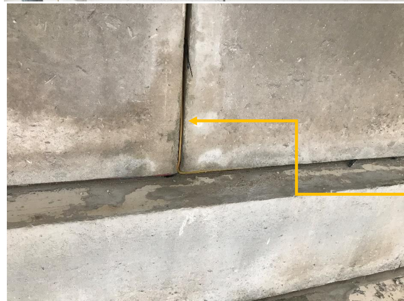
Widened masonry joints forming a chase before anode installation
