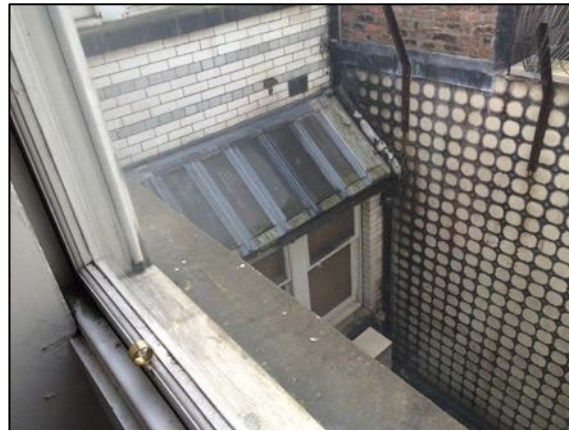
Detail 2: Typical view of the lightwell to No. 48 King Street. Note the glazed grey brick headers.
