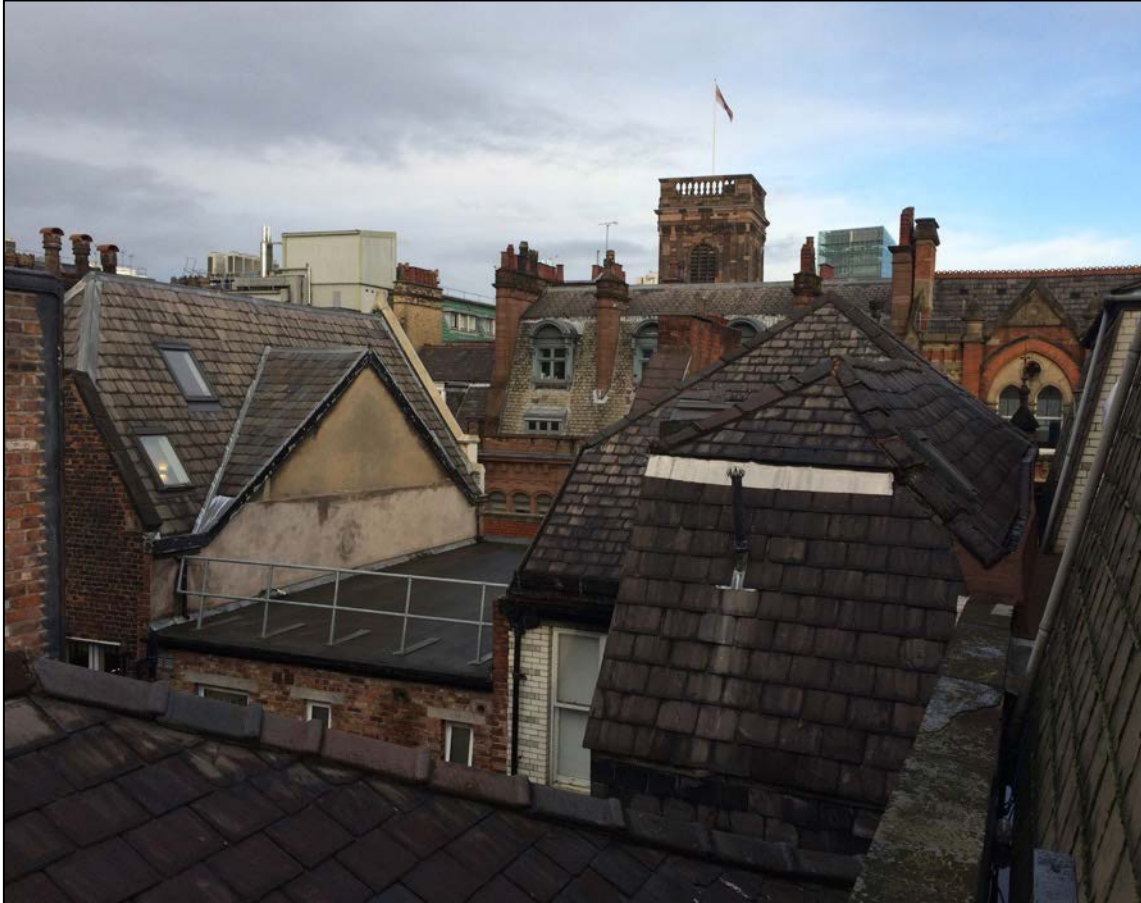
Plate 1: Roofscape looking across No. 48 King Street and the St Ann's Square Conservation Area, with St Ann's Church in the background. Note the thick cut natural slates to the roof of No. 48, and the chamfered slating detail to the right-hand side of the building to accommodate a change in level.
