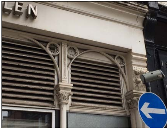
Detail 1: Surviving decorative cast iron detailing to shop front at rear of No. 48 King Street (No. 37 South King Street).
