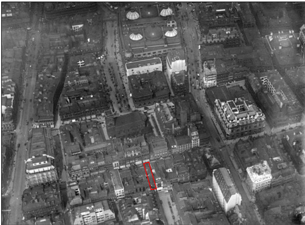
1927: Aerial view looking north-east across Manchester City Centre. No. 48 King Street can be seen towards the base of the image, highlighted in red. Whilst few details are discernible at this distance, the slate roofs and lightwell of No. 48 can be seen. (Historic England).
