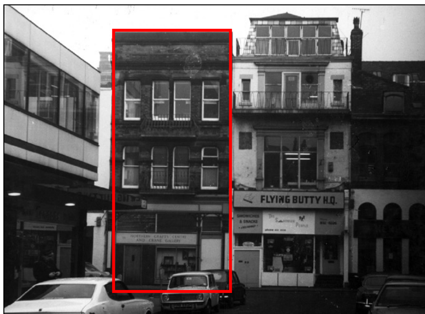
1973: The same view 13 years later shows a change in the character of the area, the “Boutique Renee” on the ground floor of No. 50 having been replaced by the “Flying Butty” sandwich bar. The ground floor of No. 48 remained in use as the Northern Crafts Centre and Crane Gallery. Part of the tower of St Ann’s Church can be glimpsed to the rear left of No. 48. (Manchester City Archives).
