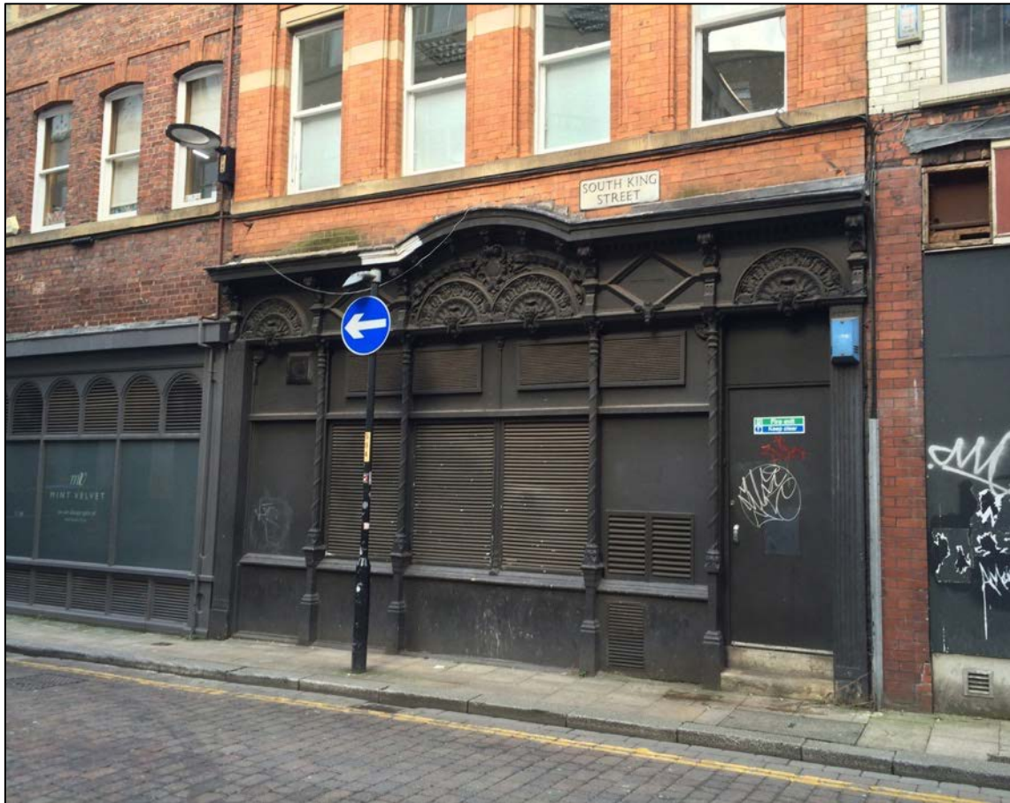
Plate 4: Typical survival of disused 19 th century shop front to South King Street, with extensive and intricate cast iron decorative detail comparable to the examples surviving to the rear elevation of No. 48 South King Street.
