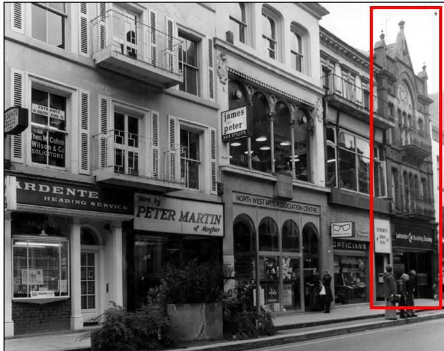
1975: King Street, with No. 48 King Street visible to the right-hand side of the image. King Street was established as a prosperous shopping street and the ground floors of most buildings, including No. 48, had been significantly altered by this time. In terms of the survival of historic features of interest at No. 48, little was to change from the date of this photograph until the present day. (Manchester City Archives).
