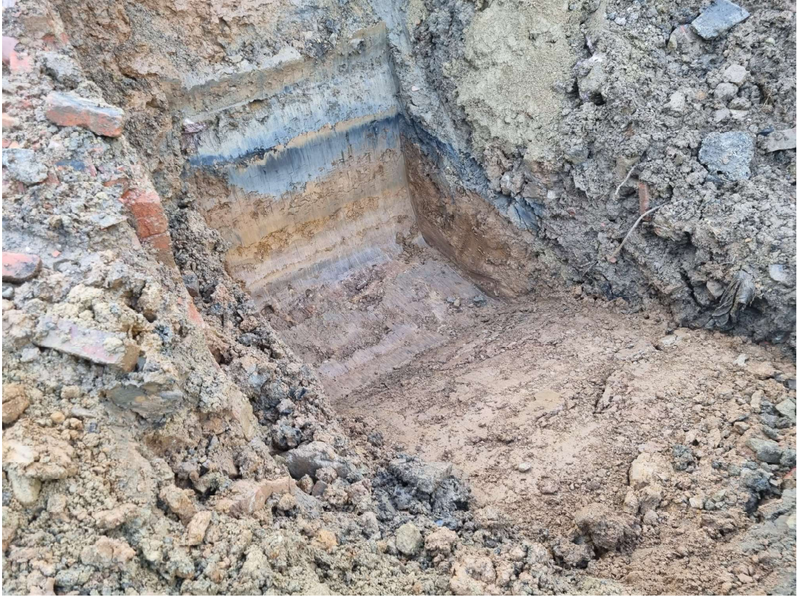
TP1 prior to testing.
