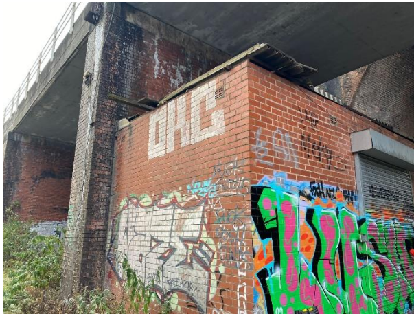
Figure 5: The brick 'hut'
