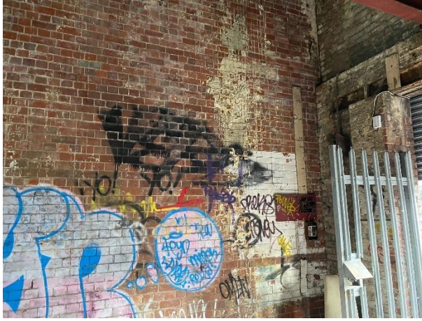
Figure 3: Plywood board fixed to the interior wall of cold store
