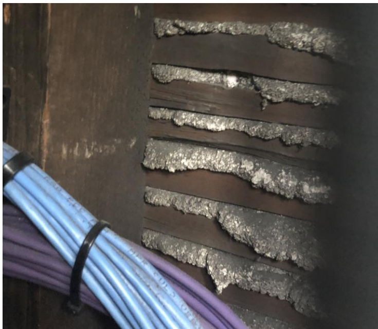
Image of reverse of laths showing plaster nibs, room 606.
