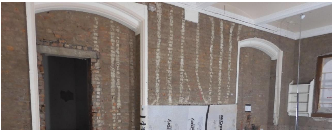
Areas of existing delaminated plaster removed from wall leaving no residue on the brickwork (note the original limewashed lines showing the route of the flues are still clearly distinct)
