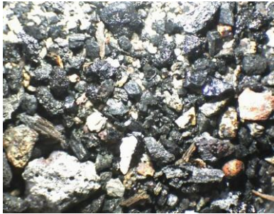
Aggregate in existing plaster mag.x10 from Hirst report 2019 showing the highly complex mix of aggregates and impurities
