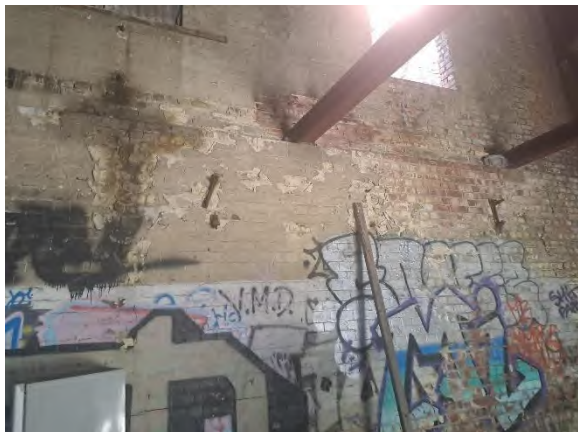
Figure 3 Internal of Cold Store Gaps by beams
