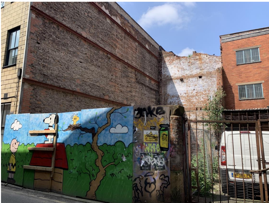
Figure 2.2: View of site enclosed by hoarding.
