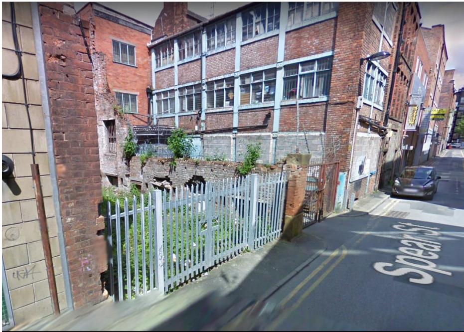
Figure 2.4: Google Streetview from 2008 showing remnants of the exterior walls of the former building on site.
