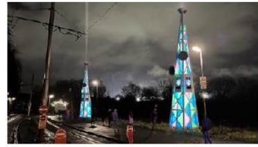
† CWT_002B - LIGHT ANTENNAS INSTALLATION
