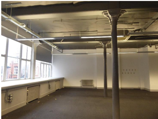
Figure 11: image of the rear of level 1 showing the large expanse of window glass and deep windowsill.
