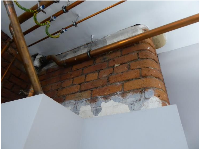
Figure 21: Section of retained historic decoration to the lower ground floor office / exhibition space.
