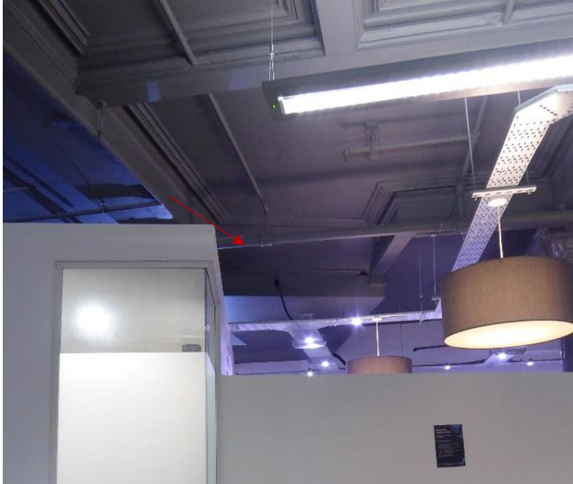
Figure 13: possible evidence of the location of an earlier staircase to level 1.
