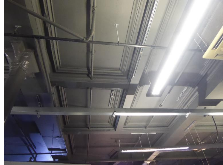
Figure 10: image of the ceiling of Level 1 showing architectural mouldings to the ceiling and beam casings.
