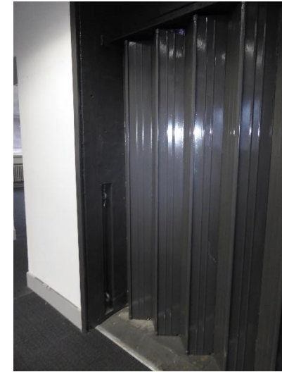
Figure 14: the former goods lift shaft to the rear space of the building.
