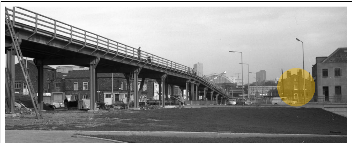
Figure 14: The construction of the new Chester Road car bridge in 1969, which was designed to carry vehicles over the newly created Mancunian Way. The southern gable end of the Former Bridgewater Canal Offices can be seen highlighted in yellow. The Site is obscured by development in the middle-ground. Source: Manchester Local Image Archive.
