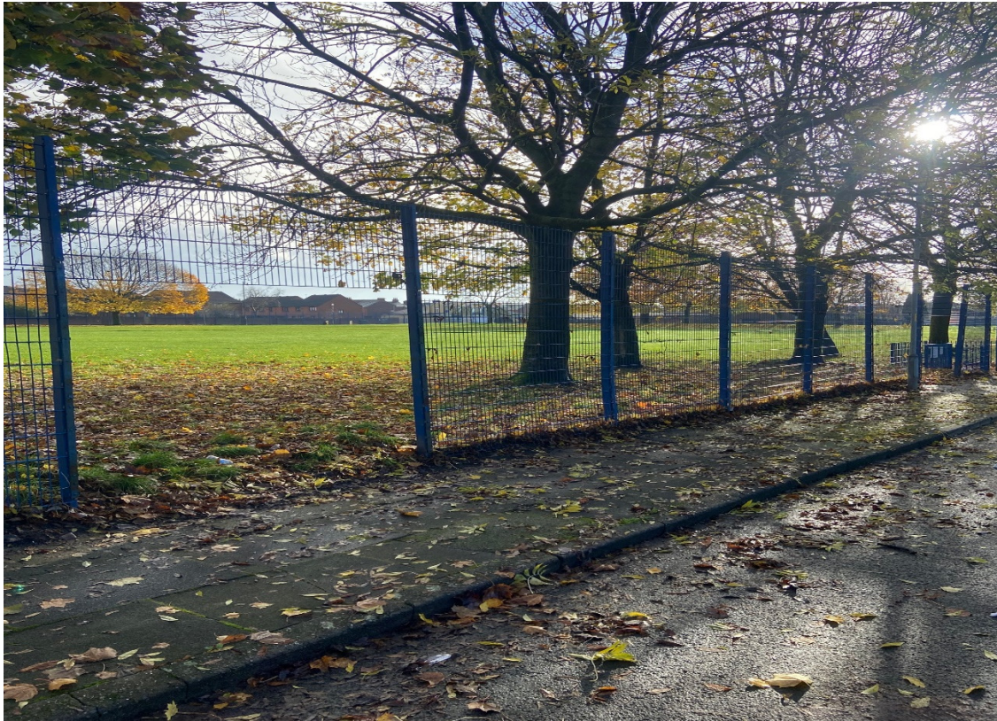
Photograph E – Image taken along Tamerton Drive facing south east, showing the blue palisade fencing running around the site with notable missing panels.
