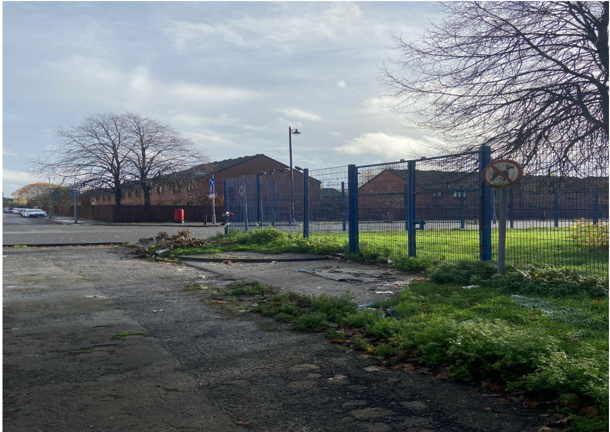
Photograph A – Image taken on Brentfield Avenue to the north of site, facing south east, illustrating the main access gate onto site for any operatives.
