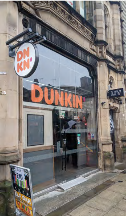
EXISTING SHOPFRONT - PHOTO
