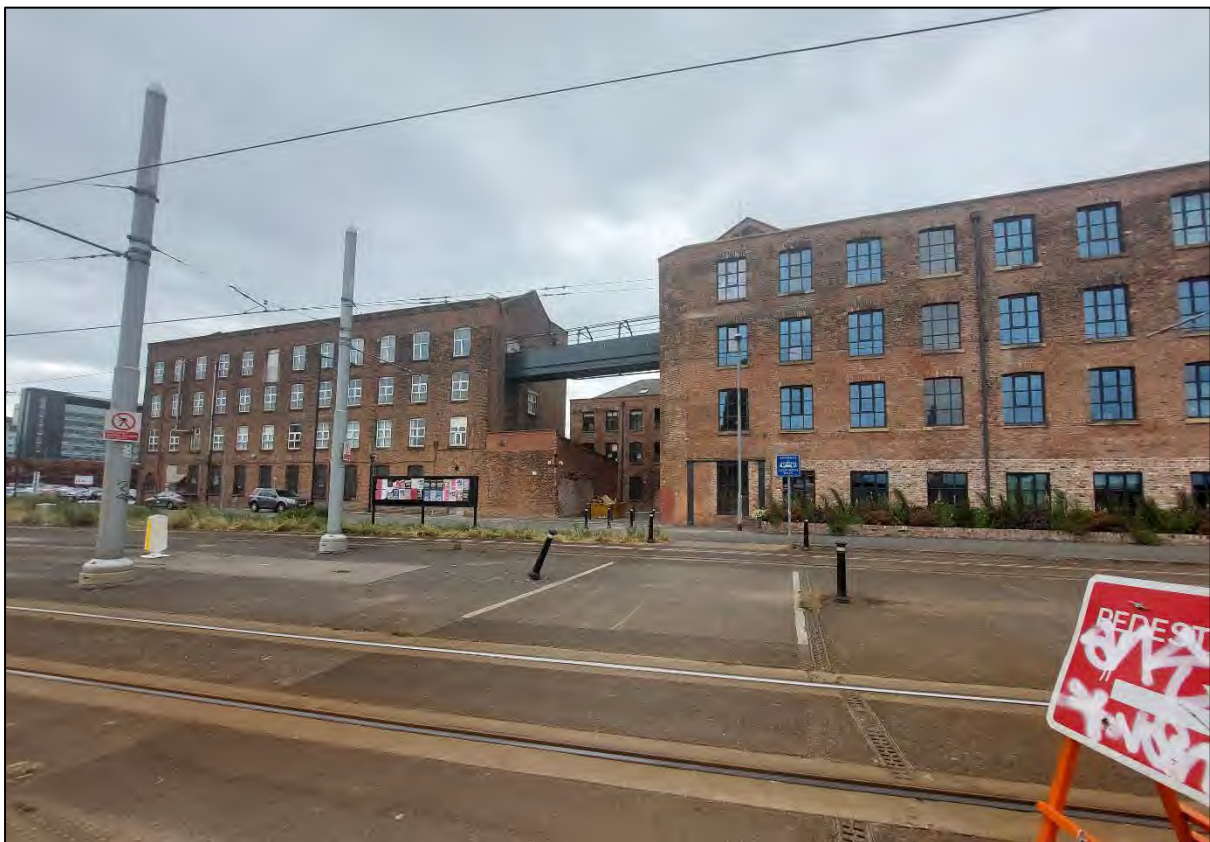
Plate 23 Alternative view of Crusader Works from the north end of Portugal Street, looking in broadly in the direction of the Site
