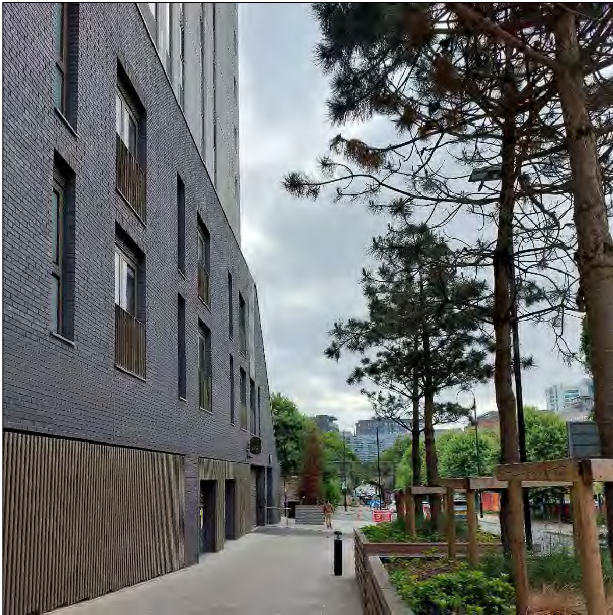
Plate 18 View of Store Street Aqueduct, looking west in the direction of the Site
