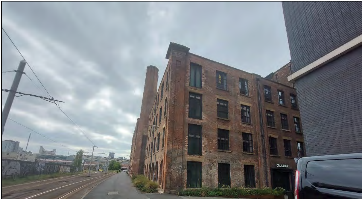
Plate 22 View of Crusader Works when looking north-west in the direction of the Site from Fair Street
