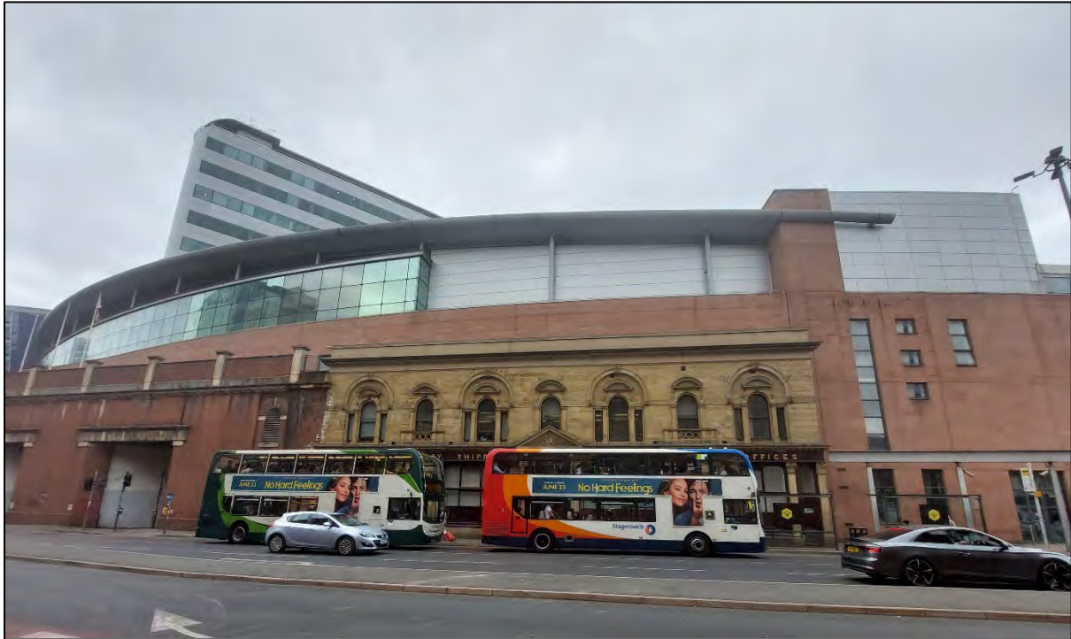
Plate 20 View of Enquiry, Delivery Shipping Cartage and Goods Agents Offices façade, looking north-east in the direction of the Site
