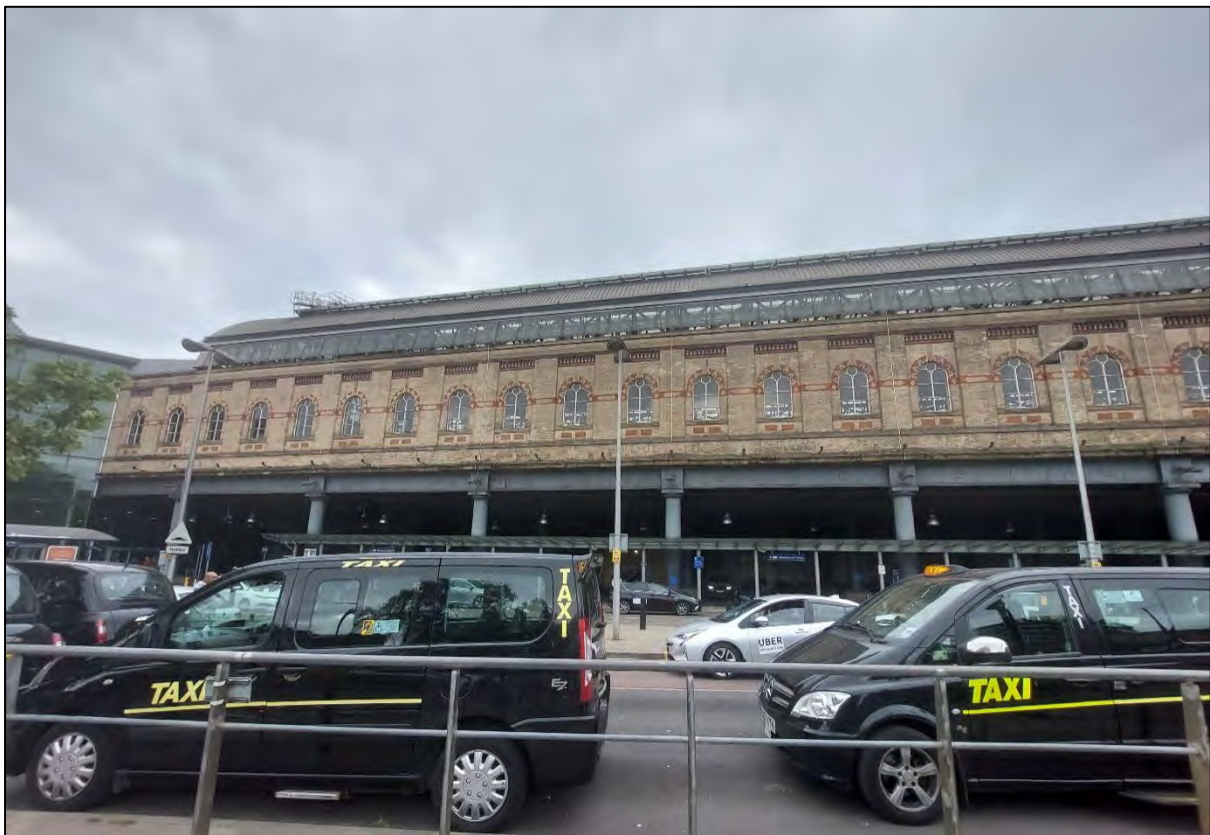
Plate 21 View of train shed looking north-east in the direction of the Site
