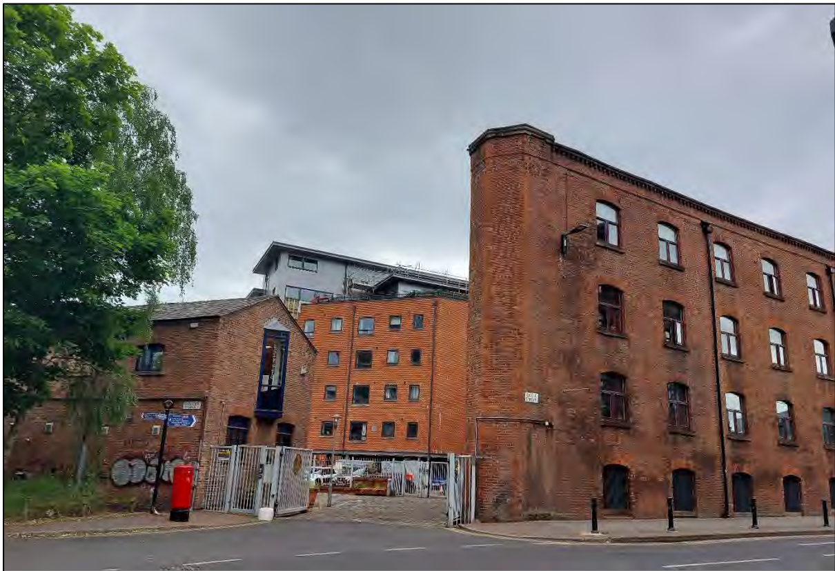
Plate 26 View of Junction Lead Mills and Stable block to south-east of Junction Lead Mills, looking south-west, in the direction of the Site
