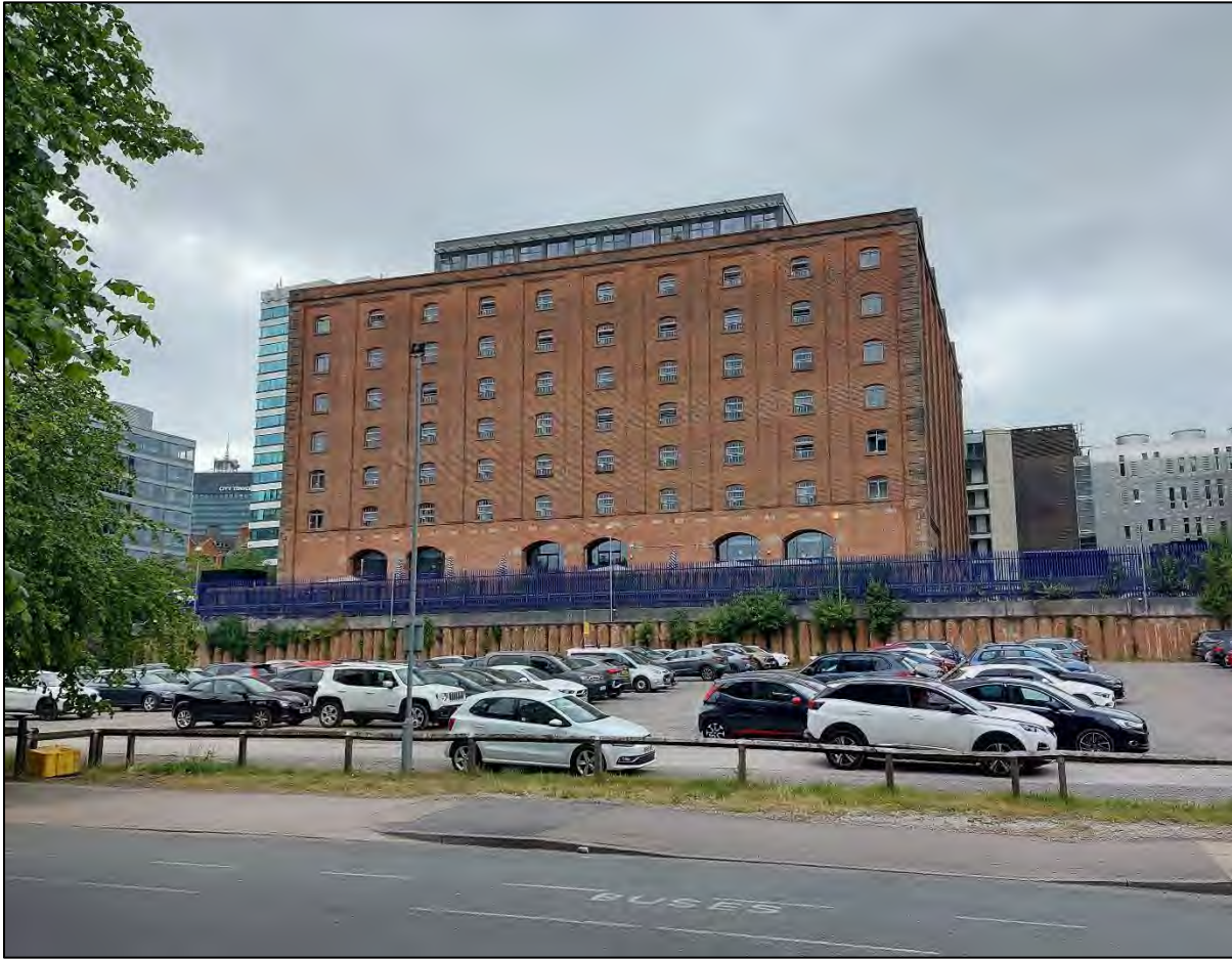
Plate 24 Key view of Ducie Street Warehouse, looking broadly north from Store Street (in the opposite direction of thew Site), showing its position raised above the Store Street street-level.
