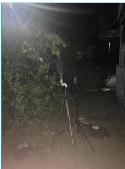
Figure 3 – Installed Noise Logging Equipment
