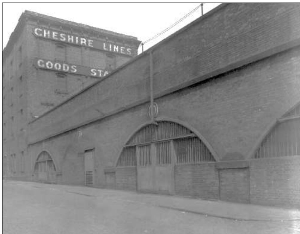
Figure 11: Watson Street Railway Arches to the northern end of Watson Street in 1938. The arch frontage is shown to have formally comprised large sliding doors on transom head rails and vertical iron bars (since removed). Note: The arches which comprise the extant Site are not shown in the image.
