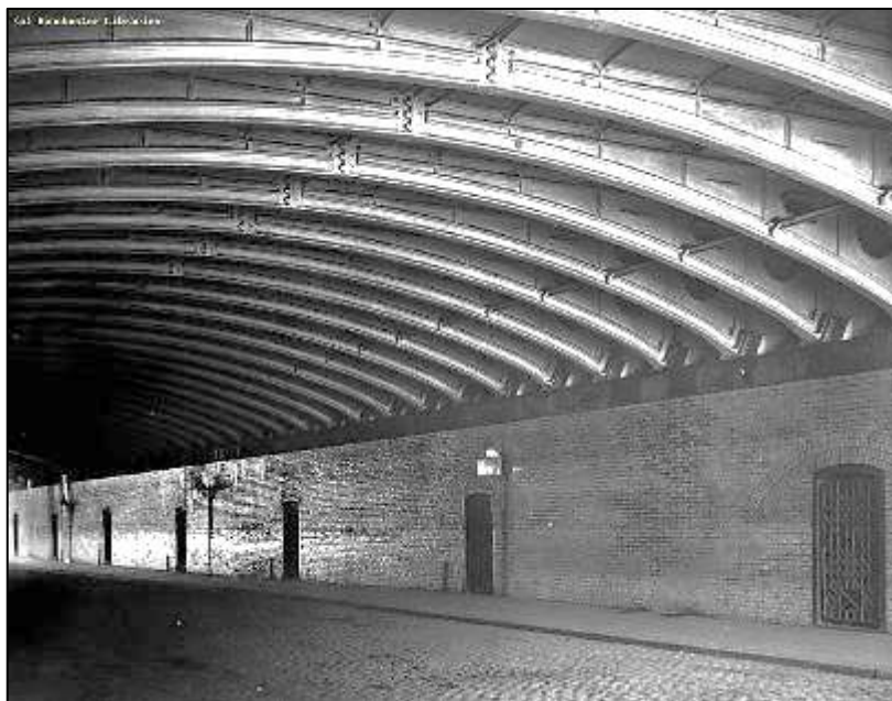
Figure 9b: (1910s) Direct access onto Great Bridgewater Street was permitted from No.19. The doors as shown in the image to the left (1905) were set within white glazed brick walls, which remain largely unaltered. The original cast-iron roof structure beneath the 1870s viaduct is also evident on the image, shown as it appears today. Source: Manchester Image Archive.
