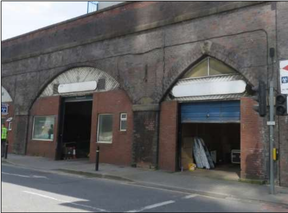
Figure 15: Image of extant site following the 1980s refurbishment works to the frontage. Note the removal of iron bars and large doors. New brick; cladding; single pane windows and roller shutter doors. Source: Site Visit, July 2019.
