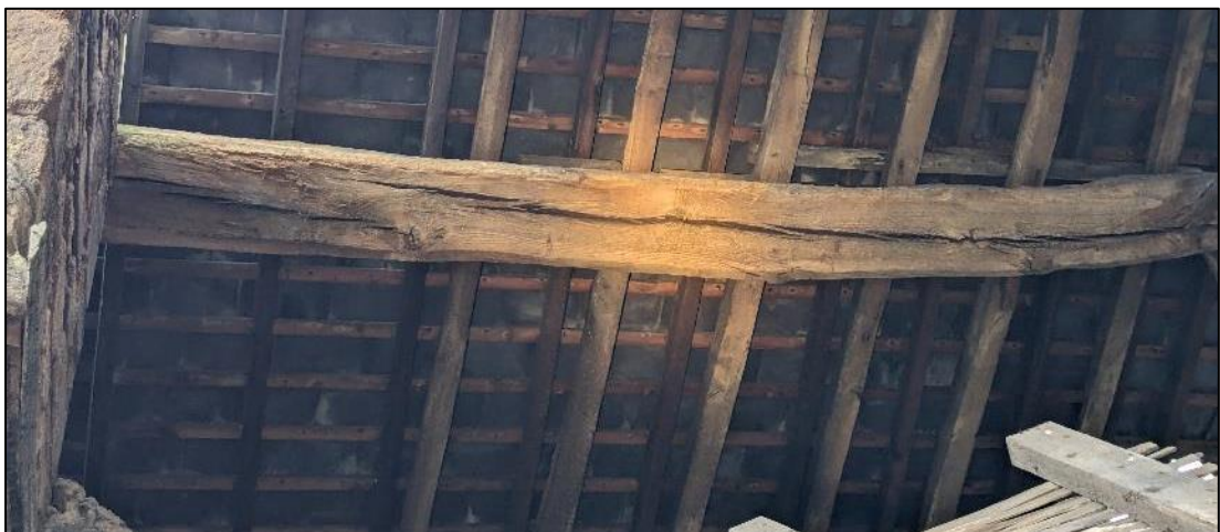
Plate 6. Desiccation fissures/cracks in purlin
