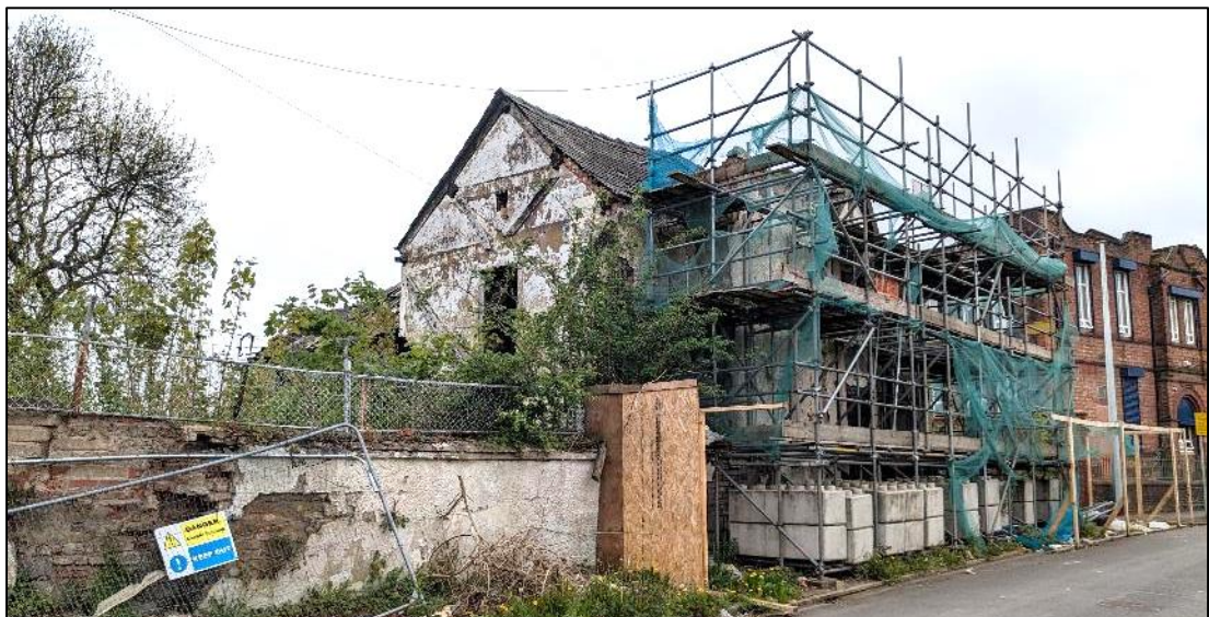
Plate 1. Northeast elevation of Hough Hall, enclosed by scaffold
