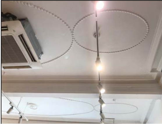
13. Ceiling decoration scheme within ground floor shop floor bays adjacent to King Street.
