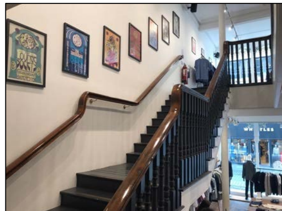
24. View up principal staircase towards first floor from dog leg landing.
