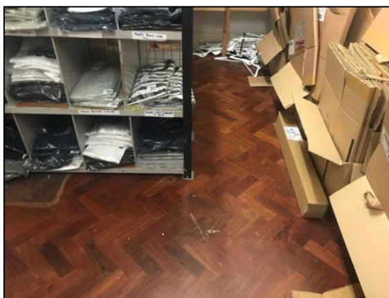
11. Typical section of timber parquet flooring within basement.
