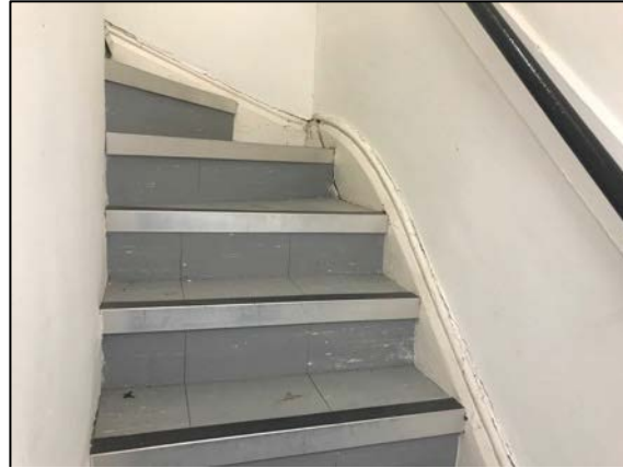
26. Typical example of original timber skirting board within rear secondary staircase.
