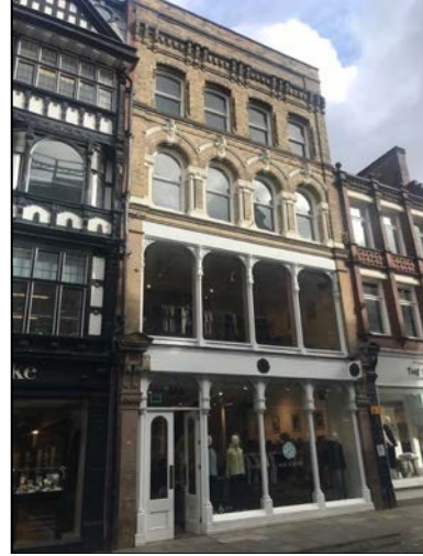
2. Main south elevation of No. 19 King Street. Note the unusual use of yellow Gault bricks.
