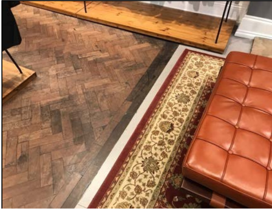
19. Timber parquet flooring to front section of ground floor.
