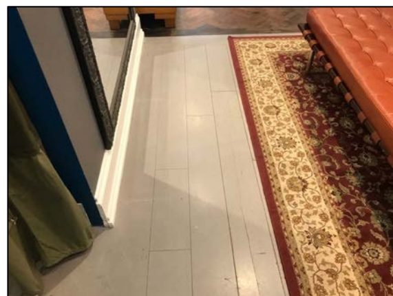
18. Typical section of traditional timber floor boards to rear section of ground floor.
