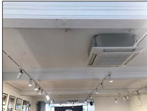
28. View of first floor ceiling with decorative cornices to enclosed structural beams.
