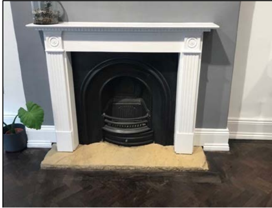
31. Rear fireplace to first floor shop floor with cast iron grate and natural stone hearth. Lightweight replacement timber surround.
