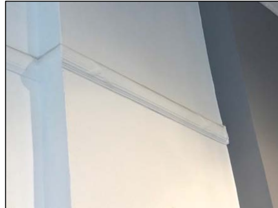
16. Detail of decorative picture rail within parts of ground floor adjacent to King Street.
