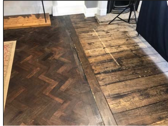
32. Detail of junction between timber parquet flooring (left) and timber board flooring (right) at first floor level.
