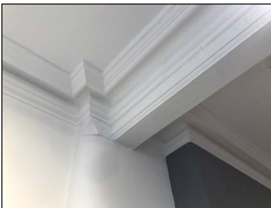
29. Detail of junction between decorative cornice to enclosed structural beam and adjacent ceiling perimeter cornice.
