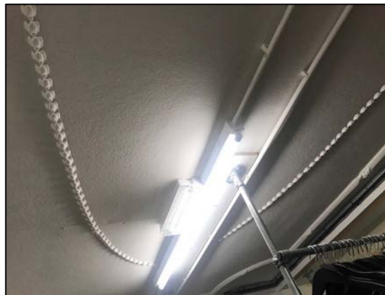
8. Typical ceiling decoration scheme within basement store area.
