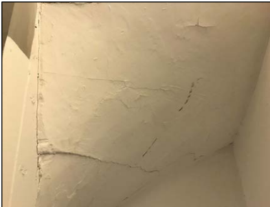
27. Typical example of original lath and plaster ceiling within rear secondary staircase.
