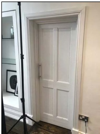
35. Original four panelled timber door to first floor fitting room.
