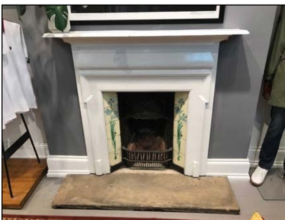
17. Fireplace with classical fire surround and original tiling with floral motif to rear of ground floor shop floor. Original cast iron grate and solid floor hearth visible.
