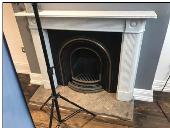
30. Rear fireplace to first floor shop floor with cast iron grate, stone surround and natural stone hearth.
