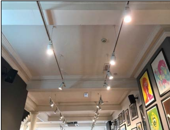
15. Typical view of ceiling within ground floor, with decorative cornice to structural beams.
