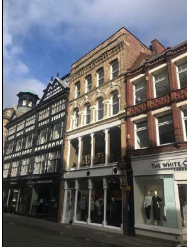
1. Main south elevation of No. 19 King Street, with Nos. 13-17 King Street (left of image)
