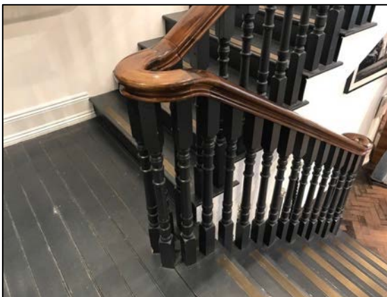
23. Detail of principal staircase at dog leg landing.
