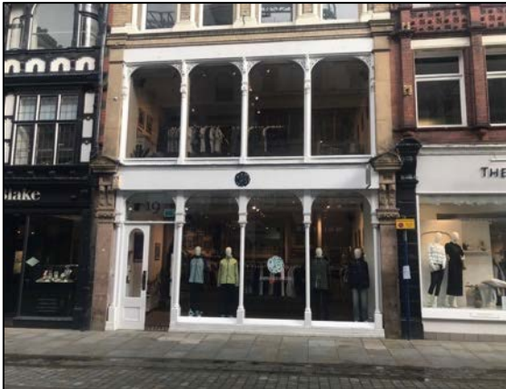
3. Ground and first floor shop front windows. Note the decorative slim cast iron columns.
