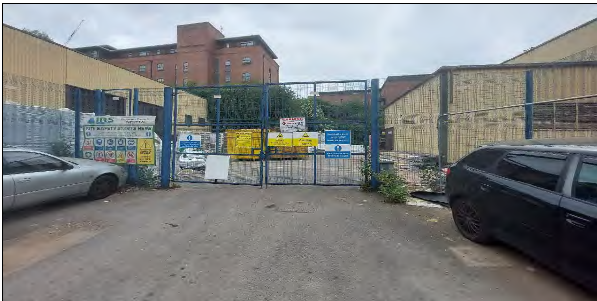
Plate 16 View of the Site looking south from Store Street
