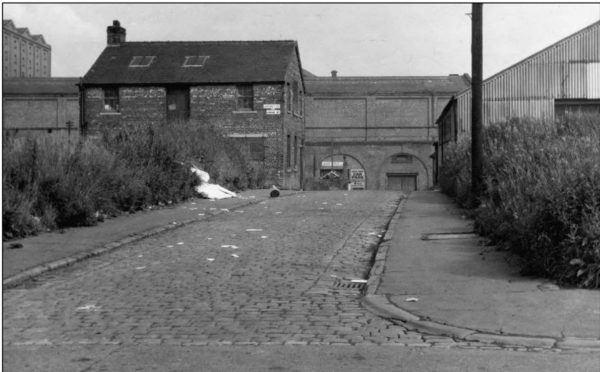
Plate 12 View of Sparkle Street, taken from Lomas Street, looking north towards Store Street, taken in 1966, courtesy of Manchester Local Image Collection
