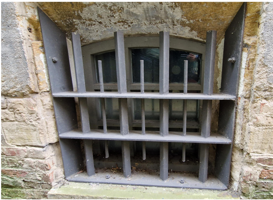
Existing External Security Bars (Nicholas Street)
