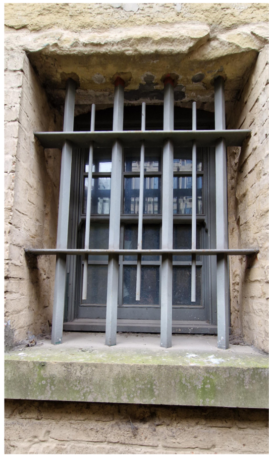
Existing External Security Bars (Princess Street)
