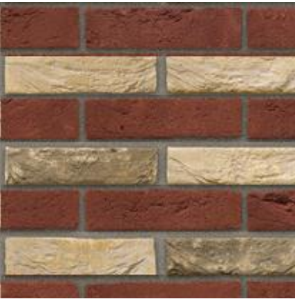
Red and Buff Banded Brickwork
