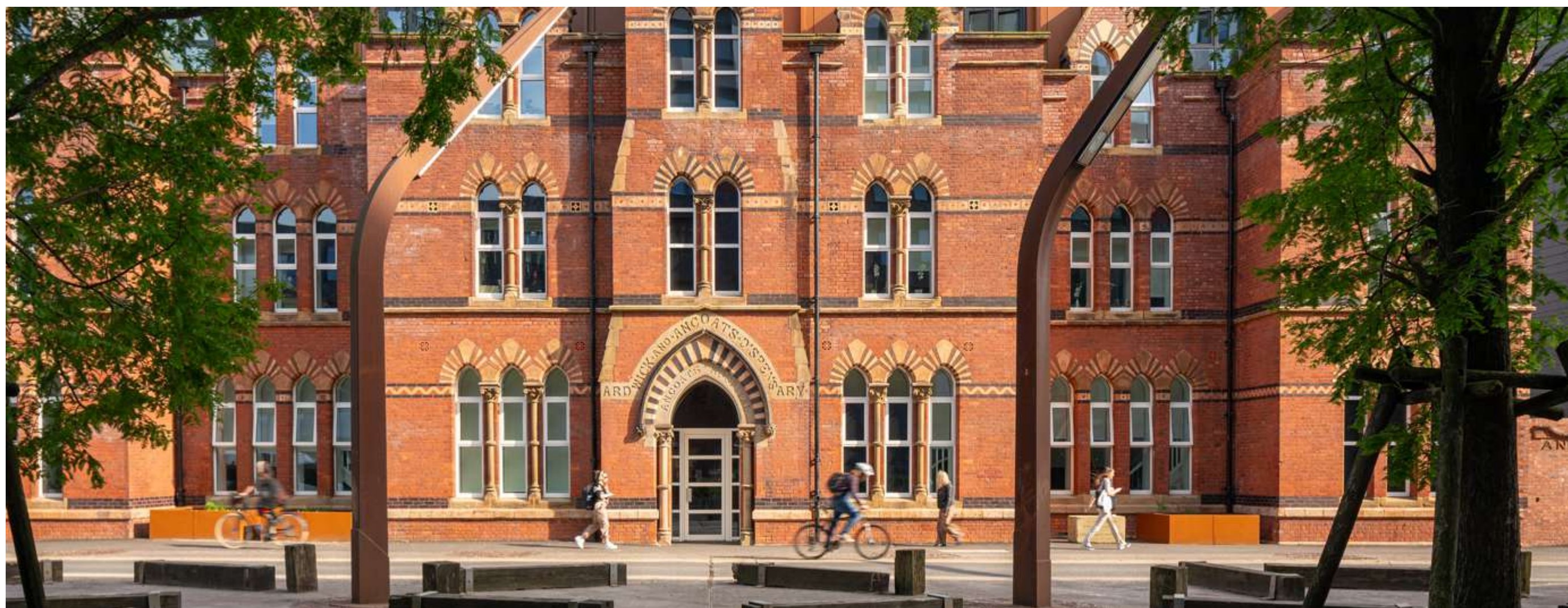
PHOTOGRAPH SHOWING PLANTER & FOUNDATION STONE IN RECESSED BAYS
