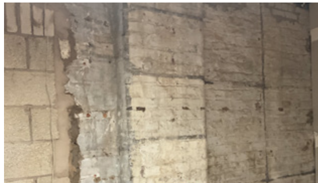
3.98 No. 21, main store, brickwork to the dividing wall with no. 23
