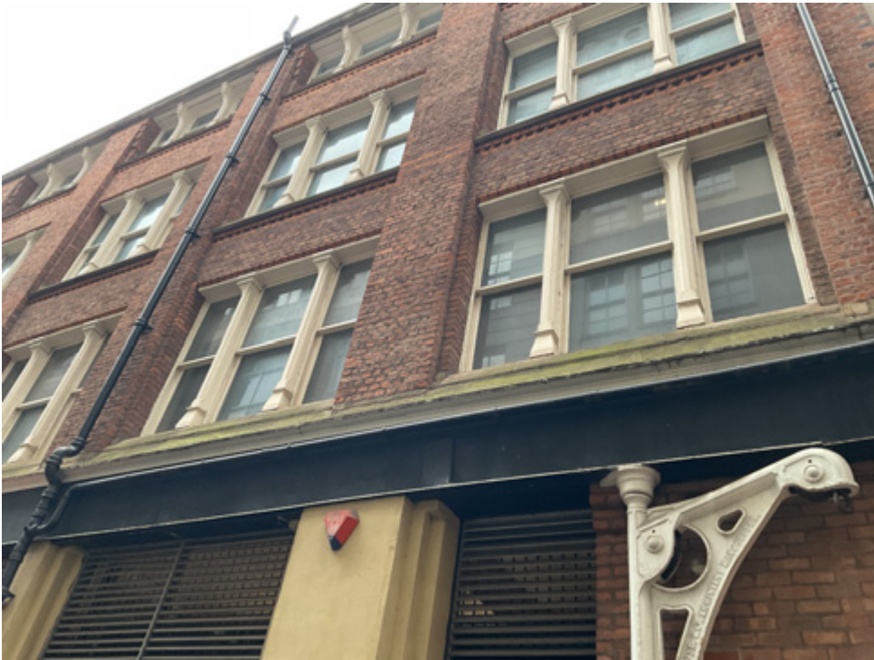
3.17 Secondary frontage, upper (office) floors
