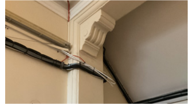
3.58 No. 21, ornamental trim and bracket to the lightwell opening
