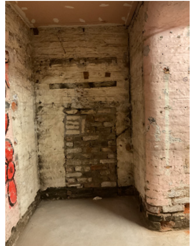
3.94 No. 21, staircase enclosure with former fireplace
