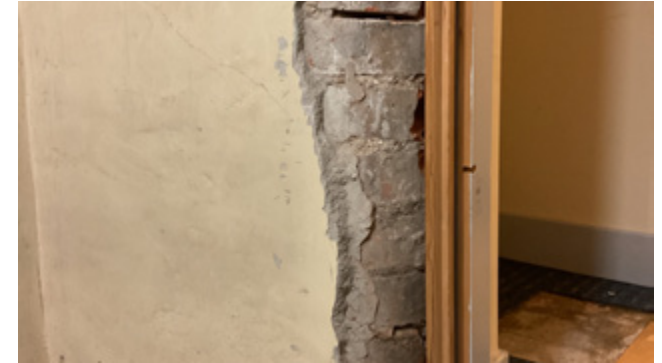
3.84 No. 17, former lightwell area, historic bricks at the base of the south wall
