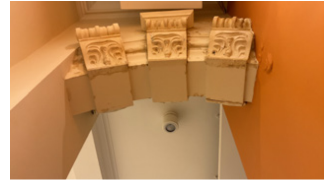
3.36 No. 17, mock stonework at the original north wall of its lightwell
