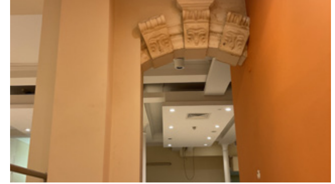
3.35 No. 17, former lightwell, the rebuilt opening with a replica bracket
