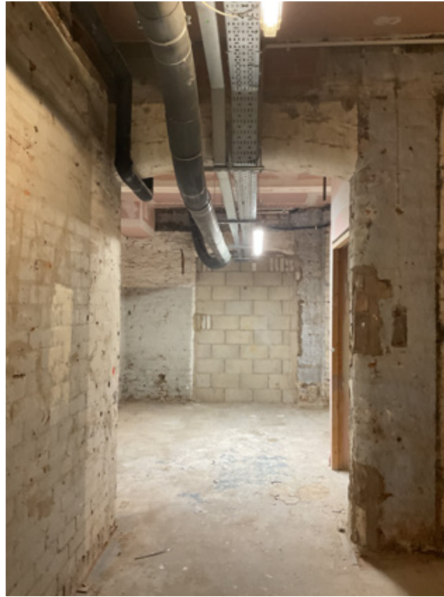
3.91 No. 19, main store, looking through the arched opening to no. 21 to the similar opening (now blocked) to no. 23
