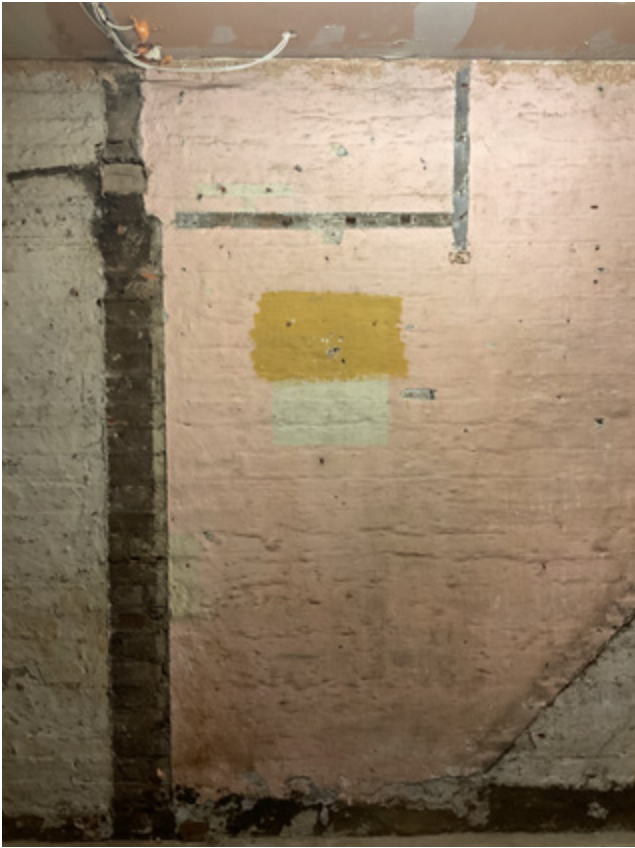
3.90 No. 19, 20 th -century south wall to the staircase enclosure, with evidence of a lost dividing wall
