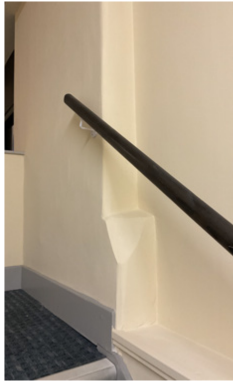
3.102 Rear, original profile of the outer wall visible adjacent to the inserted staircase
