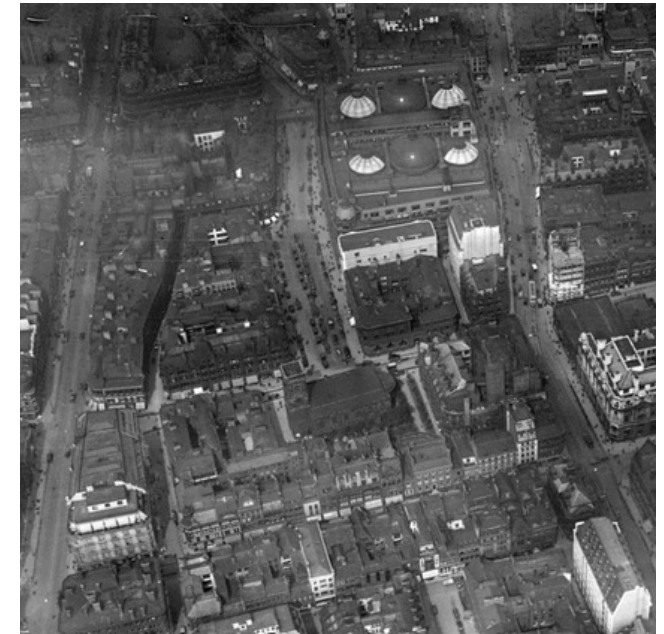
2.12 St Ann's Square and surroundings, 1927 (Britain From Above)
