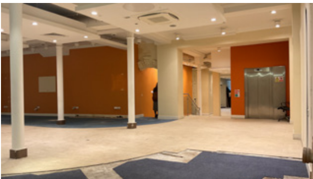
3.68 Rear, dividing wall with no. 17 (R) and former lightwell outer wall no longer aligned
