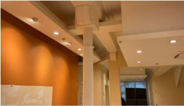
3.30 No. 17, former outer (orange) to the lightwell, the inner wall replaced by a column
