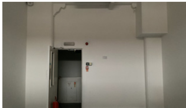
3.80 No. 23, former opening into the lightwell
