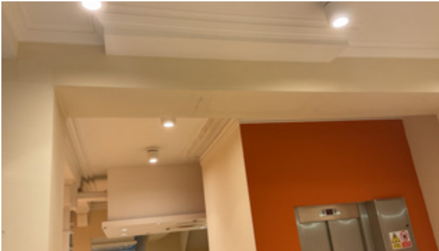
3.76 Rear, cornicing continuing around an unknown insertion to the south wall
