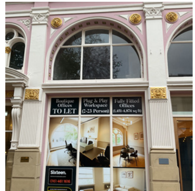
3.10 19 St Ann's Square, shopfront
