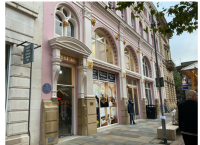
3.9 17-23 St Ann's Square, shopfronts
