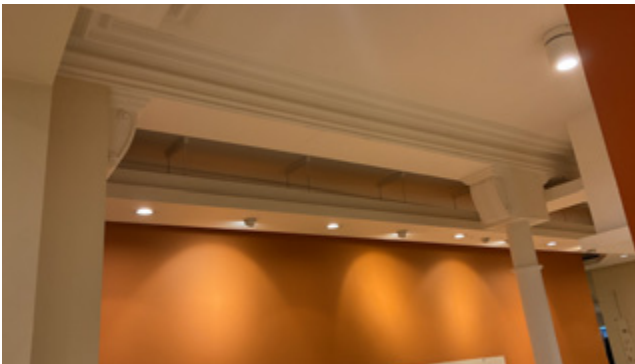
3.31 No. 17, former inner wall to the lightwell, with a later column and replica brackets
