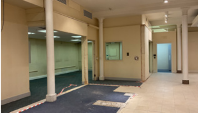
3.66 Rear, modern partitioning in the northeast and the entrance to the northeast staircase and passageway
