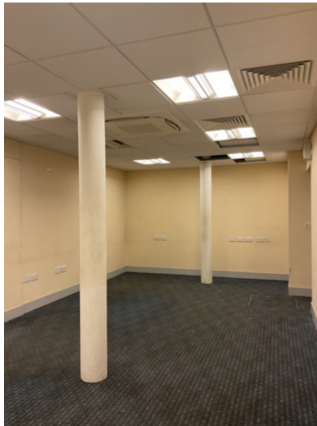
3.108 Rear, beams in the east area
