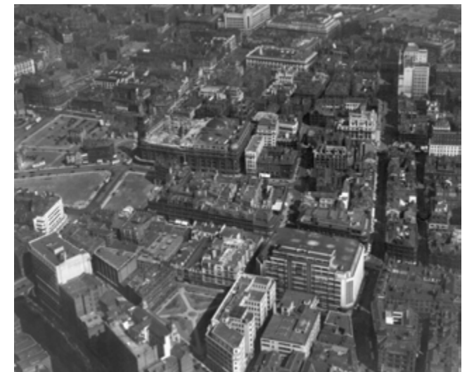
2.13 St Ann's Square and surroundings, 1948 (Britain From Above)
