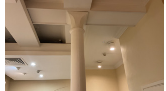
3.72 Rear, column head and coved ceiling above
