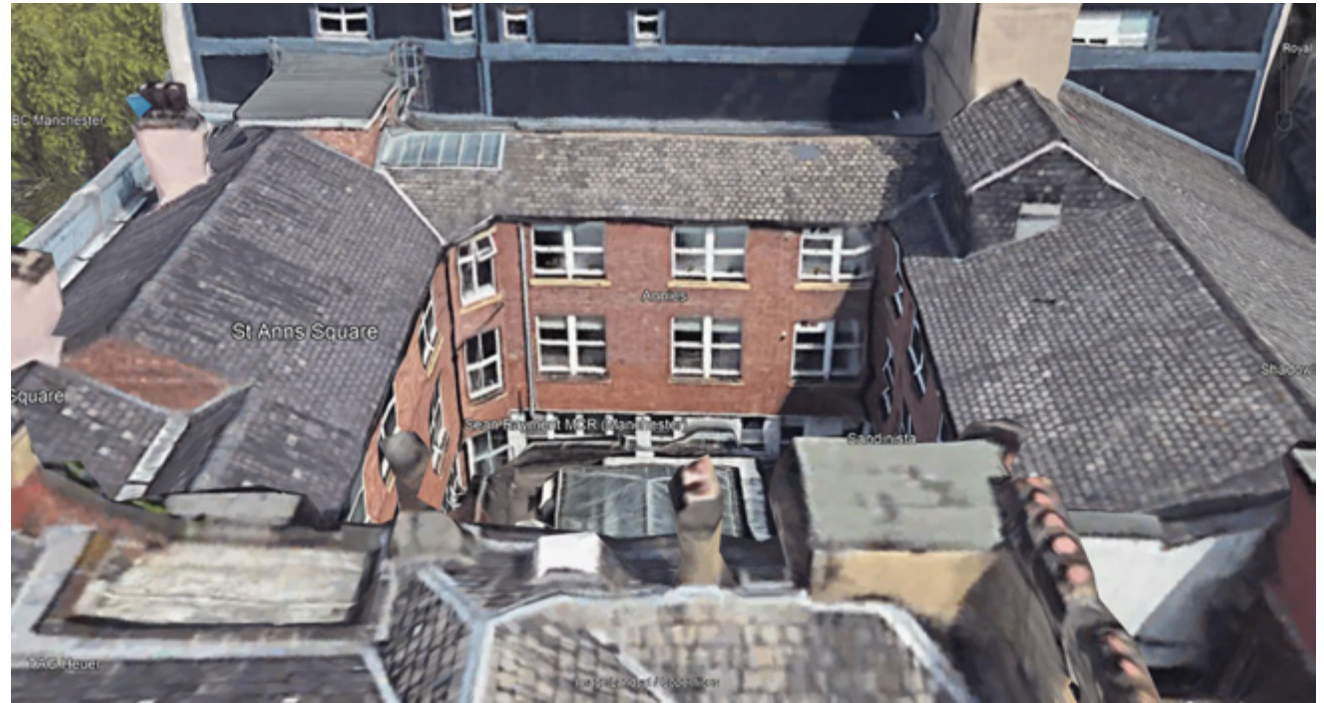
3.18 Internal elevations, 2023 (Google Earth)
