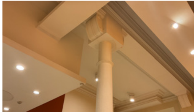
3.33 No. 17 Replica brackets to the column and wall nubbin
