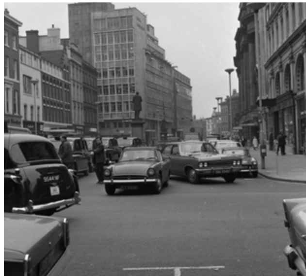
2.35 Principal frontage, 1973 (Manchester Local Image Collection)
