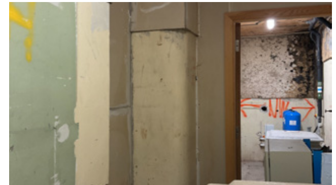
3.85 No. 17, former lightwell, stanchions along the inner lightwell wall (3)
