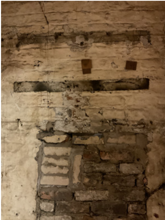
3.95 No. 21, staircase enclosure, former fireplace
