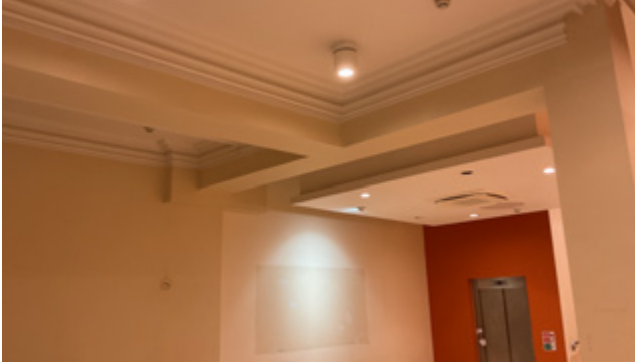
3.38 No. 17, modern inserted lift
