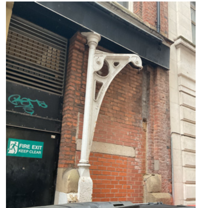
3.16 West bay, crane and former hoist location
