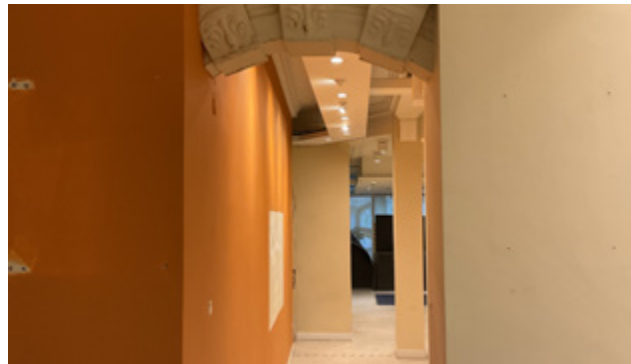
3.70 Rear, former site of the lightwell as it entered the rear (originally divided by this wall)
