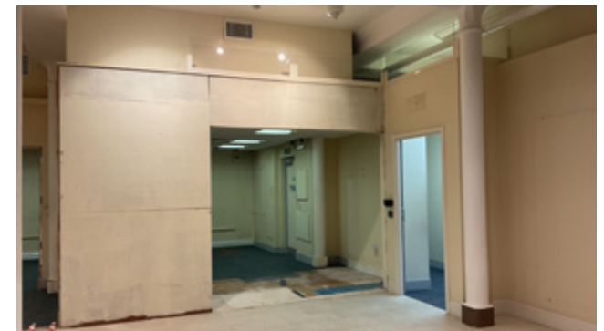
3.74 Rear, coved ceiling continuing above dropped ceilings
