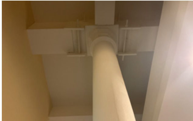
3.106b Rear, west area, exposed column head, joist and fixtures
