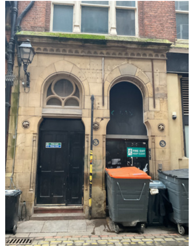
3.12 Secondary frontage, east bay
