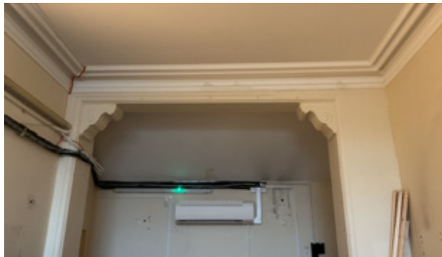
3.56 No. 21, opening to the former lightwell, with trim and brackets
