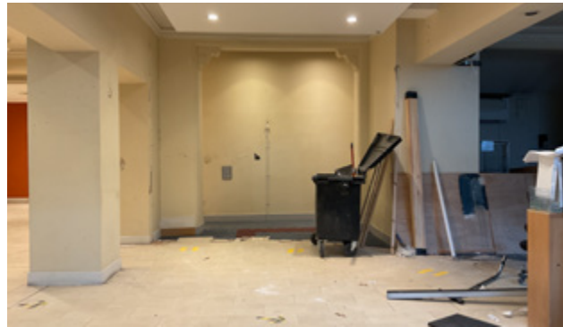
3.41 No. 19, looking north
