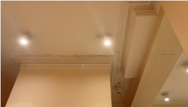
3.39 No. 17, cornicing continuing around the modern lift and an obstruction adjacent
