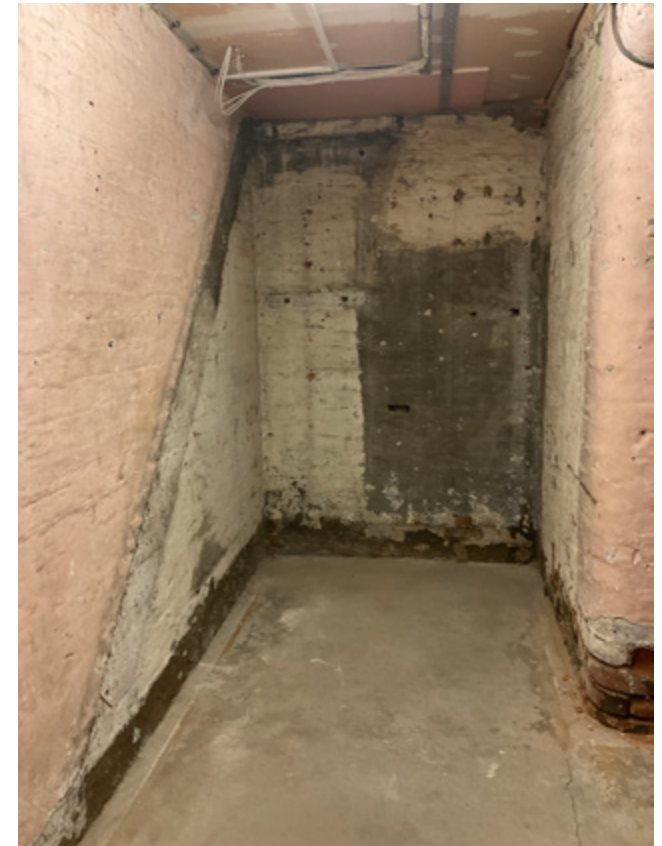
3.89 No. 19, extended staircase enclosure with evidence of a former staircase
