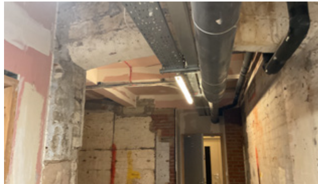
3.96 No. 21, main store, arched opening from no. 19
