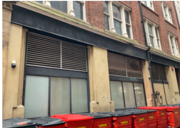
3.13 Secondary frontage, rebuilt inner bays
