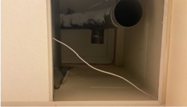
3.75 Rear, cornicing continuing above the suspended ceilings
