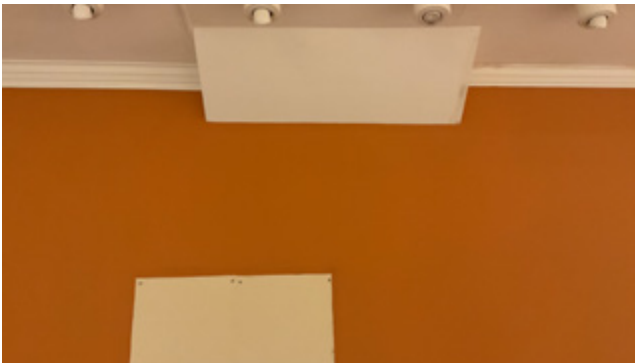
3.77 Rear, cornicing interrupted by a later insertion along the outer wall of the lightwell
