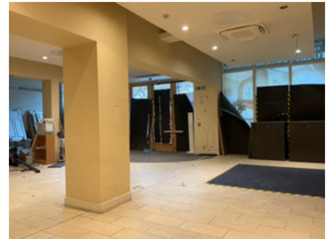
3.22 Nos. 17 and 19, remnant dividing wall
