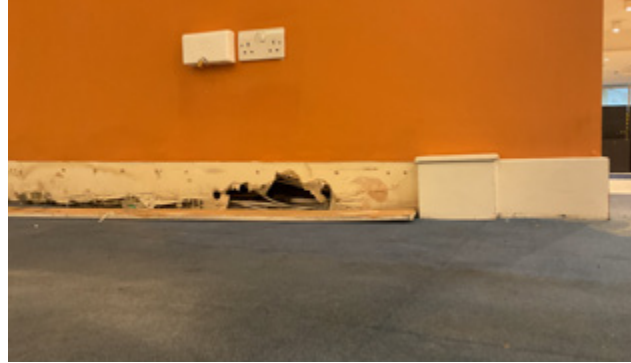
3.69 Rear, modern cabling in the south wall (former outer wall of the lightwell)
