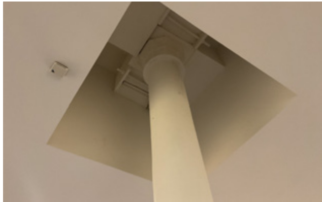
3.106c Rear, west area, exposed column head, joist and fixtures
