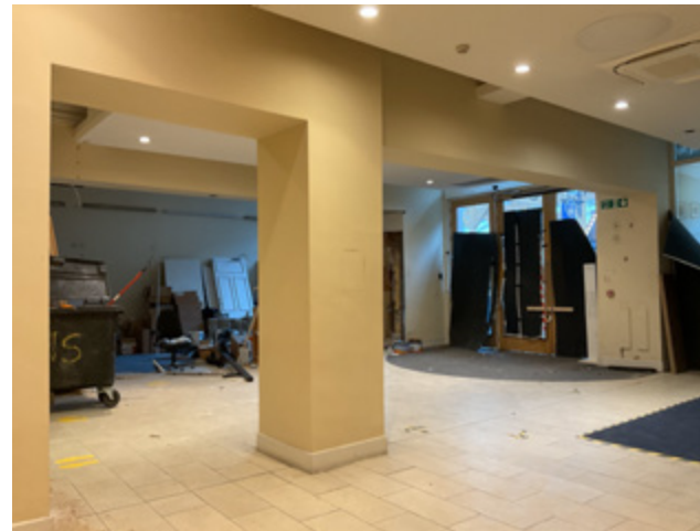
3.20 Nos. 17 (R), 19 and 21, remnant dividing walls
