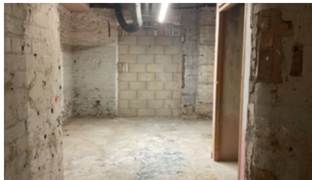
3.97 No. 21, main store (viewed from the opening from no. 19), showing the blocked arched opening into no. 23
