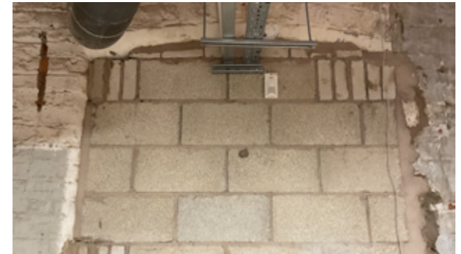
3.99 No. 21, main store, blocked arched opening to no. 23
