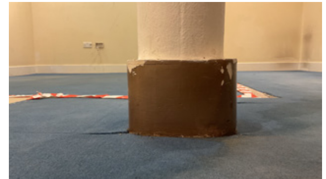
3.73 Rear, column base
