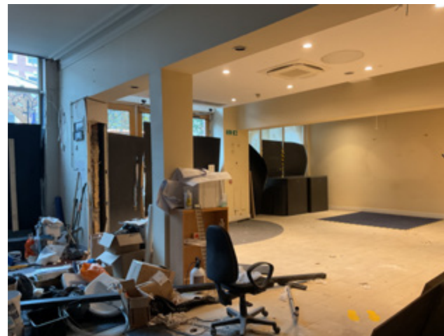
3.21 Nos. 21 (L), 19 and 17 (R), remnant dividing walls
