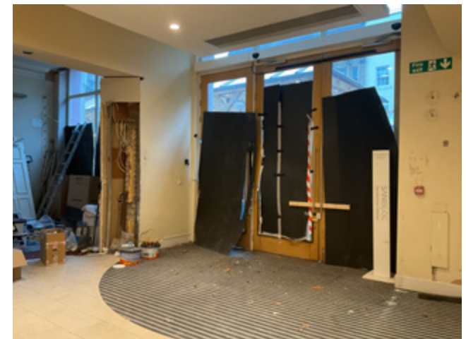
3.23 Nos. 17 and 19, dividing wall with wider plasterboard encasement
