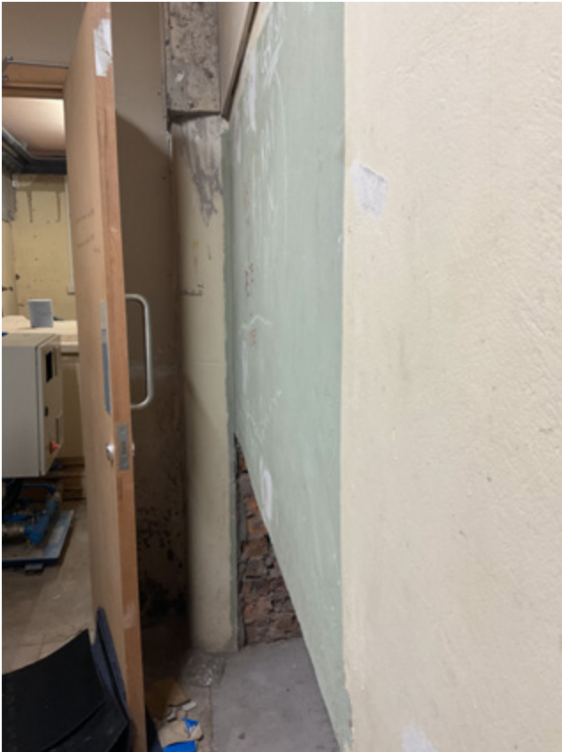
3.87 No. 17, former lightwell, stanchions along the inner lightwell wall
