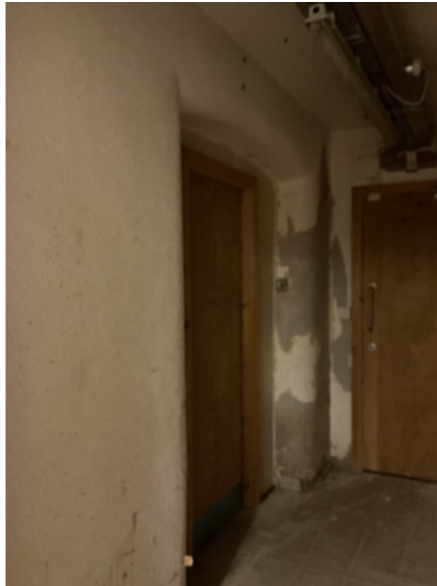
3.88 No. 19, lightwell with the arched opening into the former staircase enclosure (the modern inserted wall to the west)
