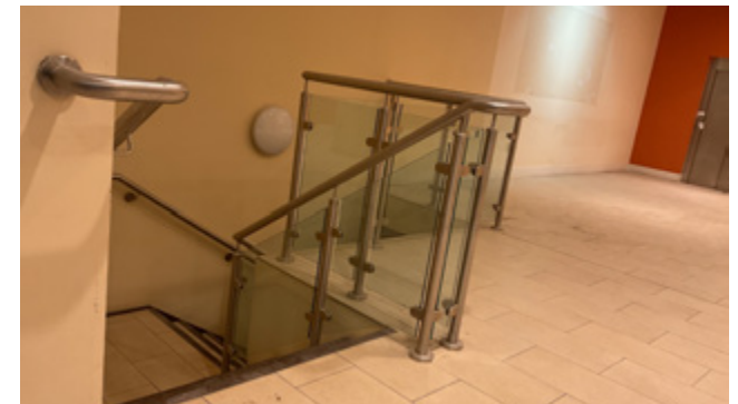
3.27 No. 17, 20 th -century inserted staircase
