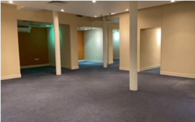
3.105 Rear, west area, columns travelling through and around the lowered ceiling
