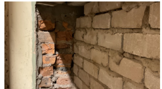
3.86 No. 17, former lightwell, brickwork to the southern stanchion of the inner lightwell wall
