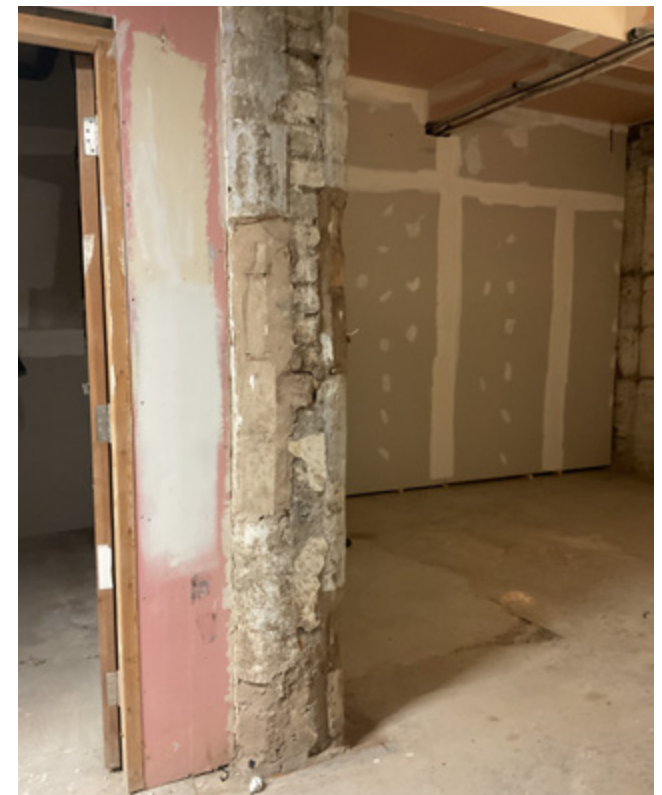
3.100 No. 21, main store, truncated partition wall
