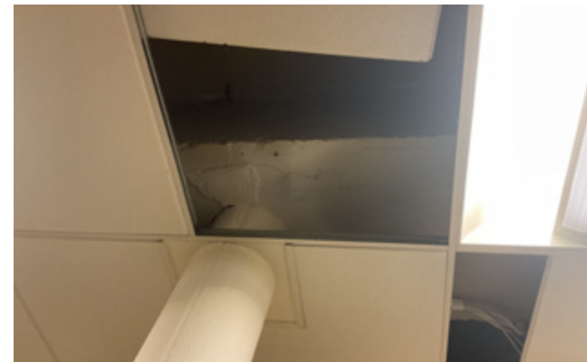
3.109 Rear, east area, columns running into concrete-encased beams
