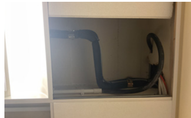
3.110 Rear, east area, underside of the floor above
