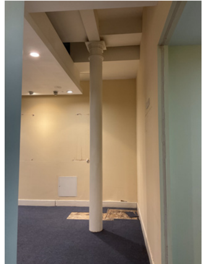
3.106d Rear, west area, simpler exposed column head
