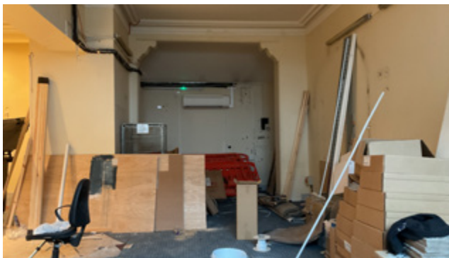
3.54 No. 21, looking north
