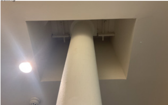
3.106a Rear, west area, exposed column head, joist and fixtures
