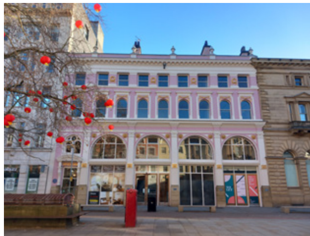
3.8 Principal frontage to St Ann's Square
