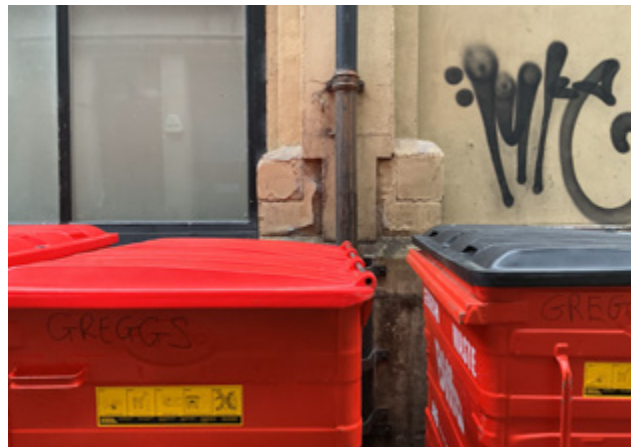
3.14 Retained structural supports
