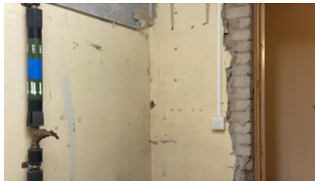
3.83 No. 17, former lightwell area, bricks in the south wall
