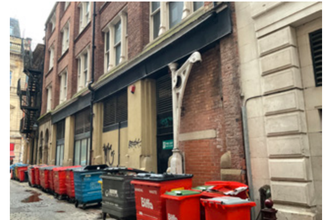
3.15 Secondary frontage, west bay
