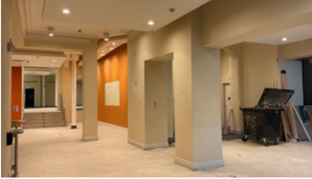
3.29 No. 17, former and surviving walls to the east
