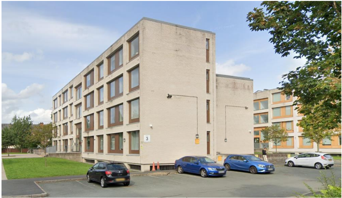
Figure 2.3: View of Block 3, with Block 2 in the background
