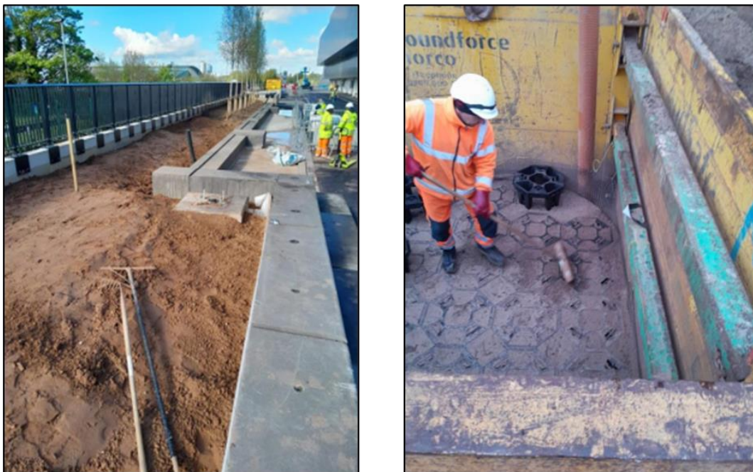
Figure 3-1 Early soft landscaping works within the public realm surrounding the Co-Op Live Arena
