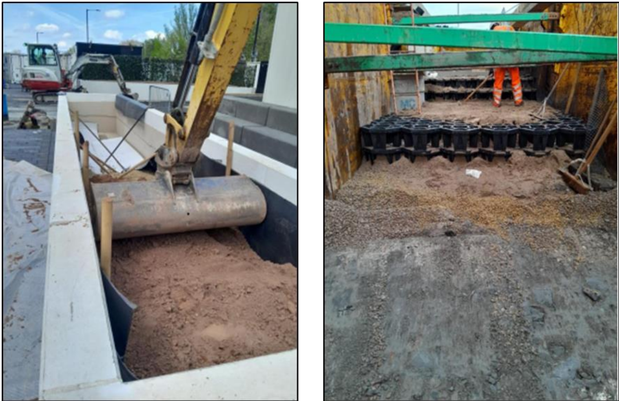
Figure 3-2 Placement of imported subsoil and topsoil
