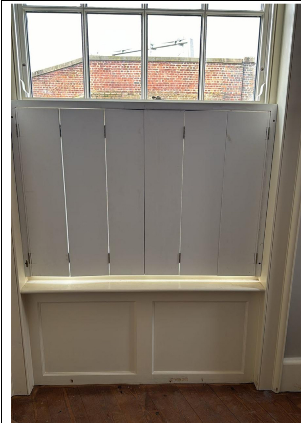
Closer view of closed shutter
