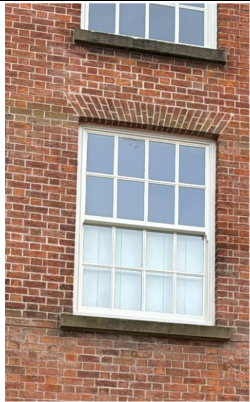
Shutter external view
