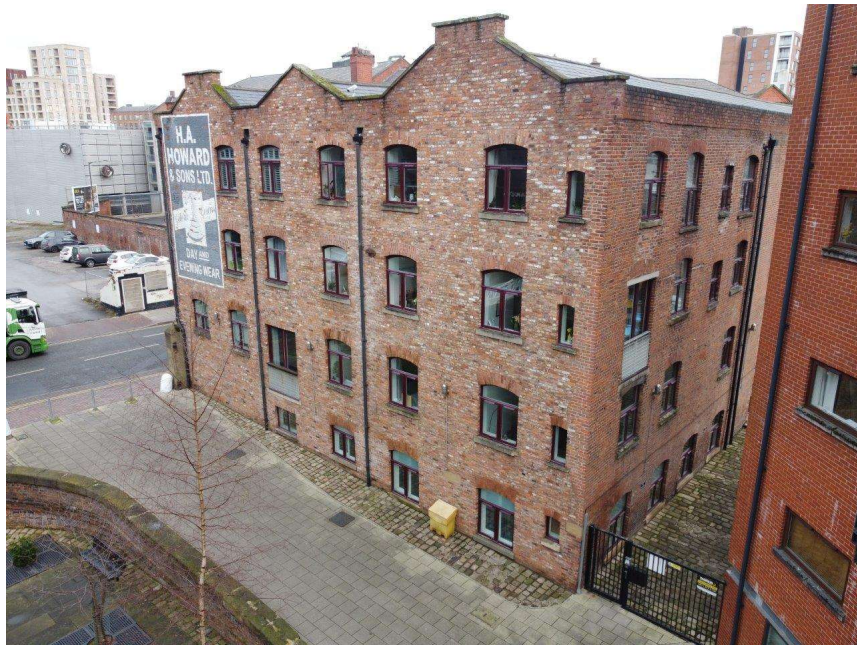
Elevation facing due Southwest
