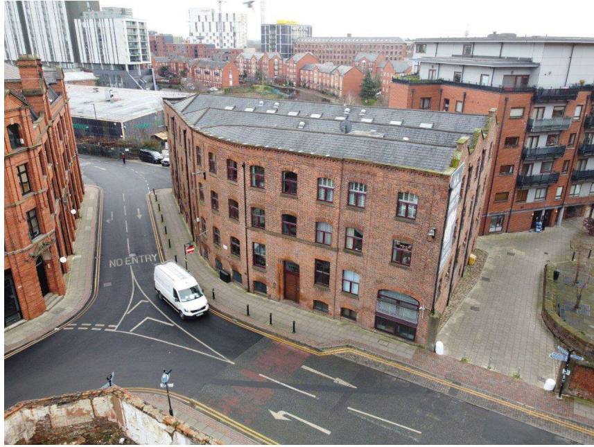
Elevation facing due North
