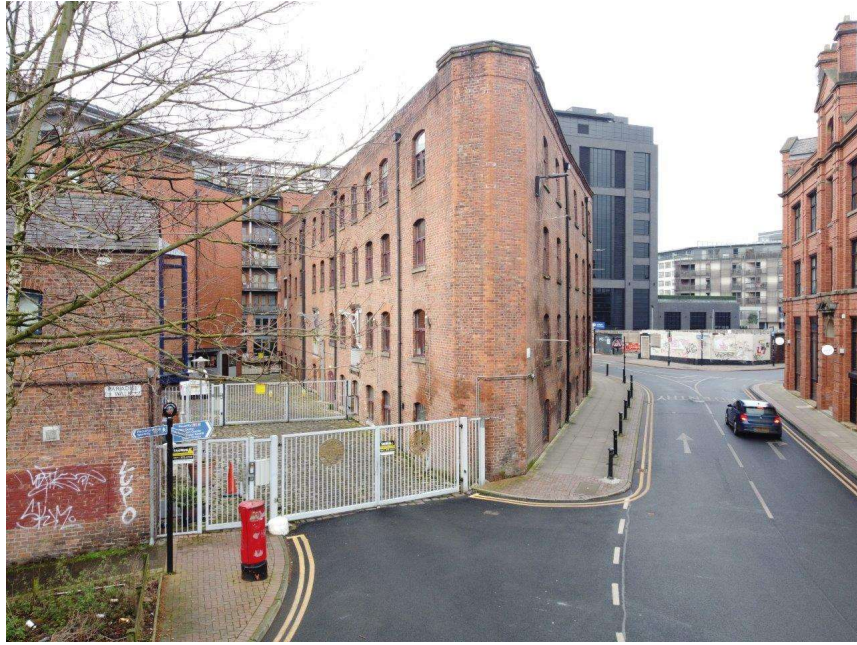
Elevation facing due Southeast
