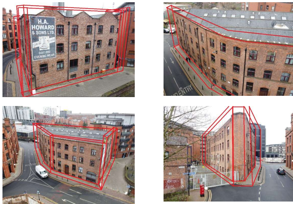
Full height scaffolding to be installed to all elevations
