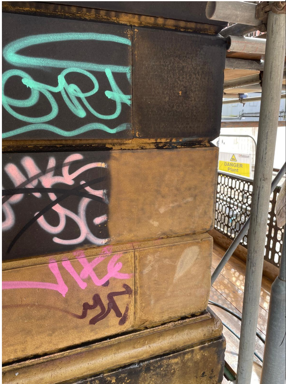
Fig 2: Nitro-morse Removed and Tensid Anti-Graffiti Ghost applied and washed off.
