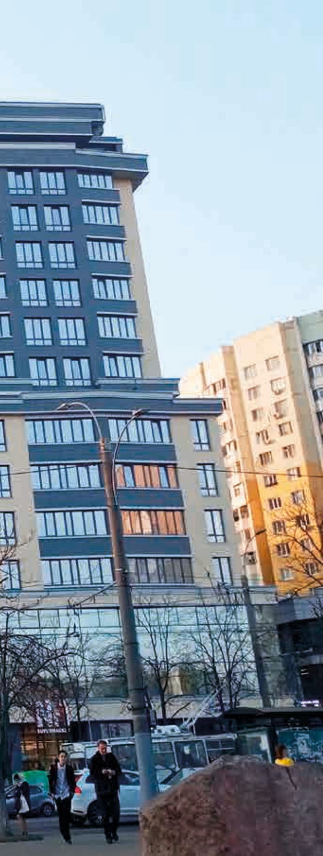
Proyecto/ Project : ParkHouse Residential Building. Chisinau (Moldova)
