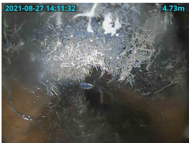
MH 8X_c7efd044-e13a-41ee-a0d0-93e8ff13e98e_20210901_145719_708.jpg, 00:00:30, 4.73 m Roots, fine
