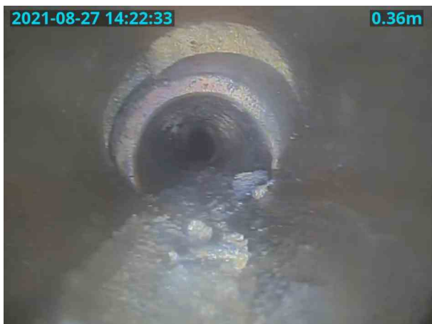
Branch AX_ad256bea-f4bc-4946-8a56-98df24e15d9c_20210831_135 028_248.jpg, 00:00:07, 0.36 m Joint displaced, large
