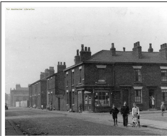
Figure 11: View from Crown Street toward the corner of Wood Street on the north-west corner of the Site, 1954. Source: Manchester Local Image Archive, Image Ref. 25952
