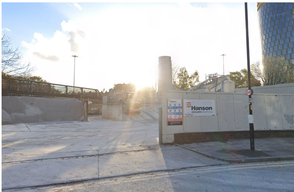
Figure 3: View into the Site from Great Jackson Street to the north-east. Source: Google Maps.
