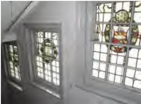
Historic photo of internal condition
