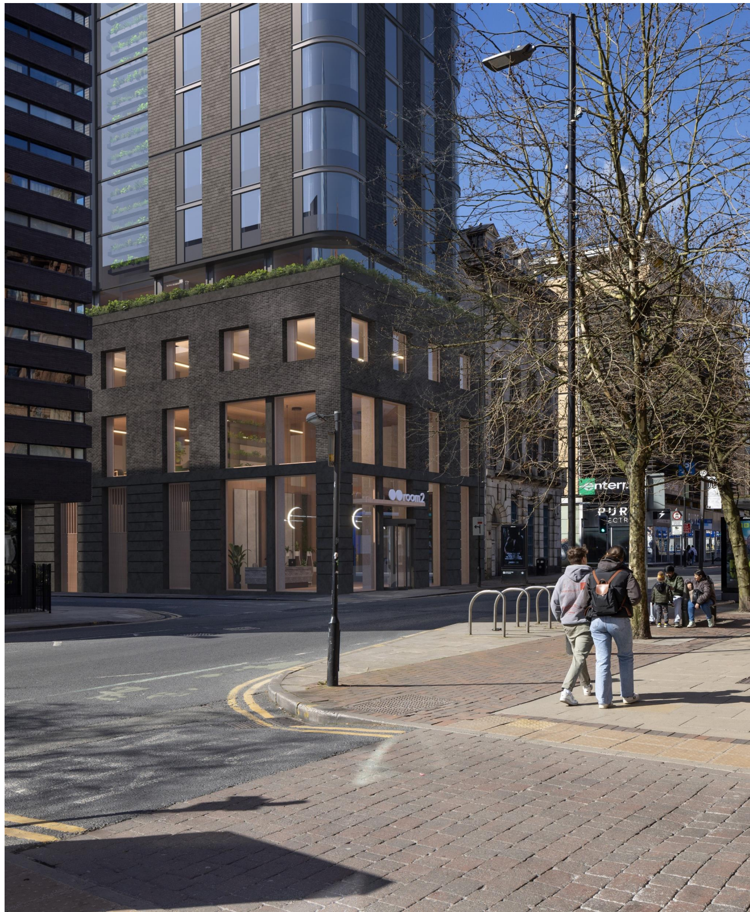
Version of submitted view with grey precast and metalwork to tower
