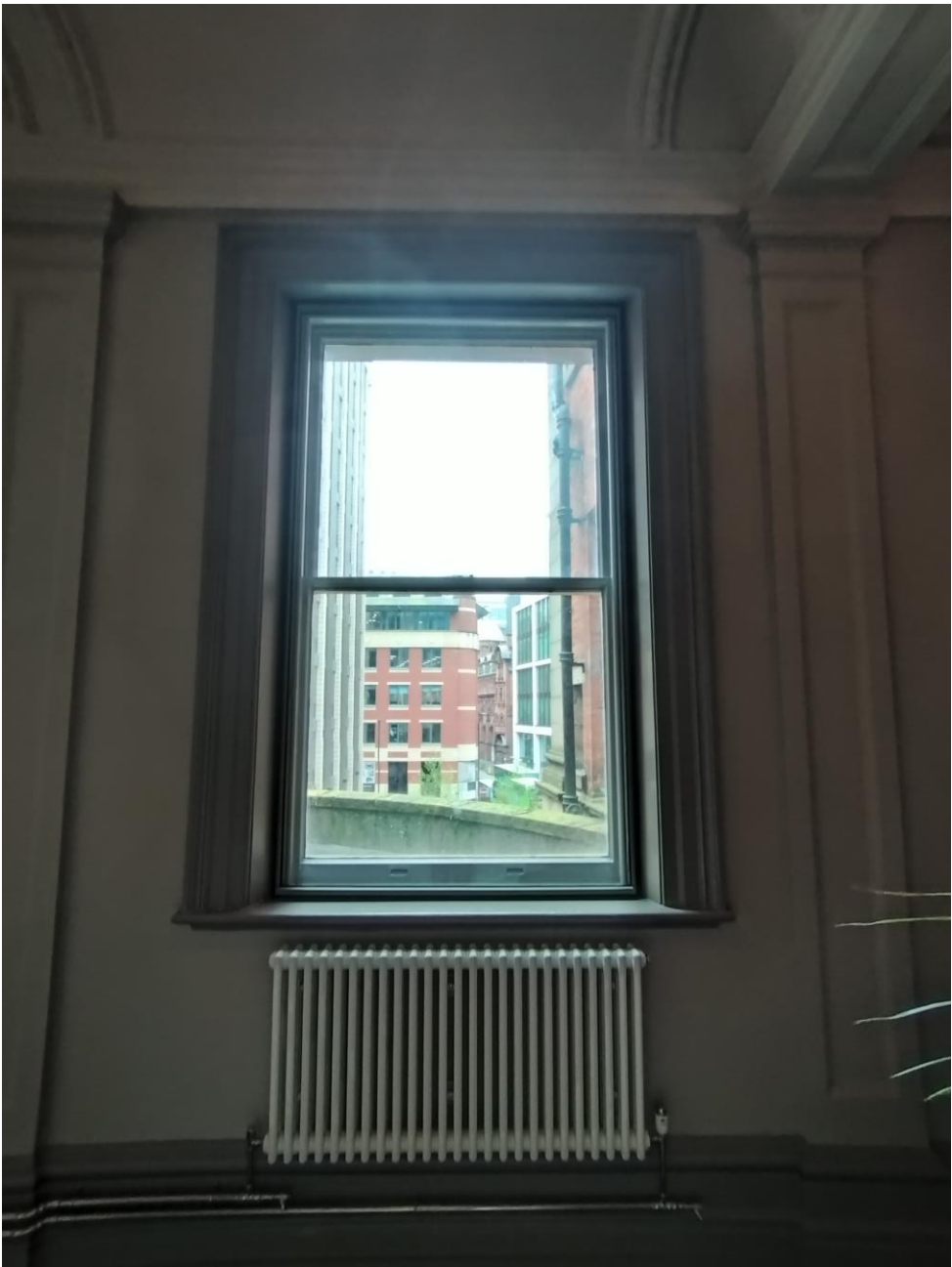
Secondary, slimline glazing system at 38-42 Mosley Street, Manchester
