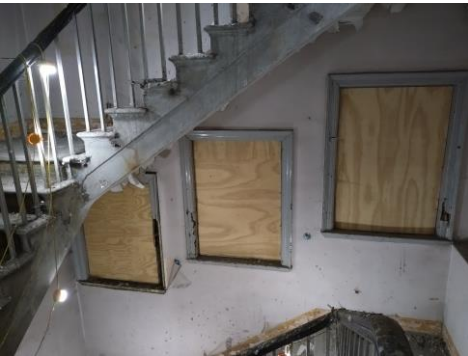
Site photographs of current internal condition of stained-glass window openings
