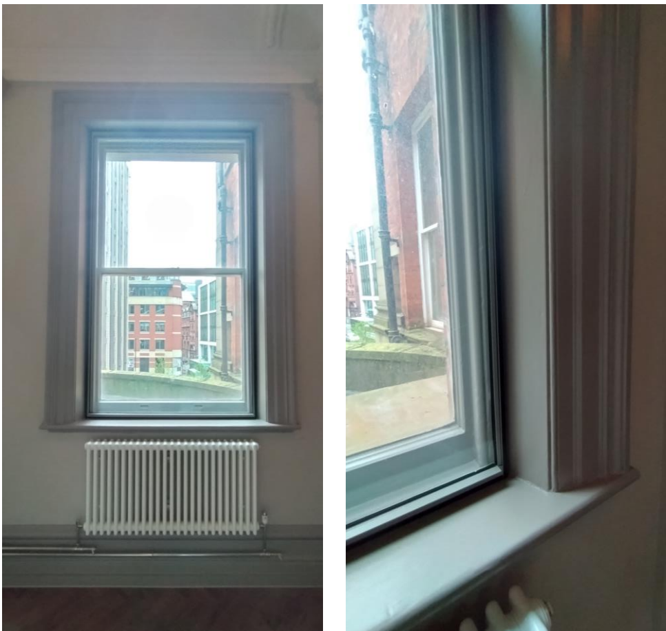
Reference images of slimline secondary glazing units used in another Grade II listed building in Manchester
