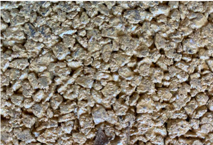
Sample of Asphalt
