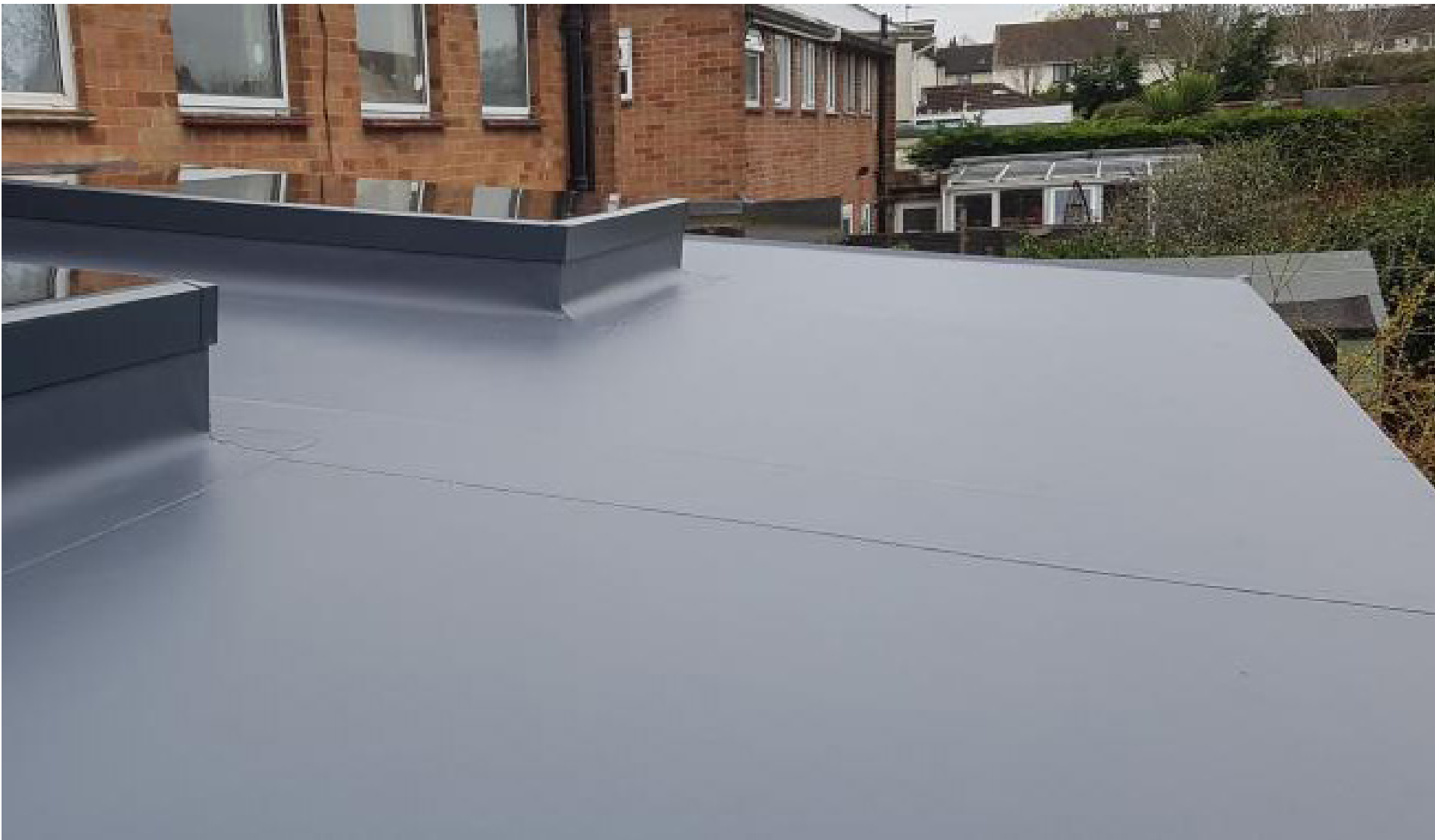
Example of Single Ply Roof
