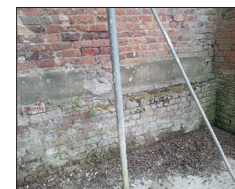
C2 - Existing brickwork wall to be retained and necessary remedial works carried out.
