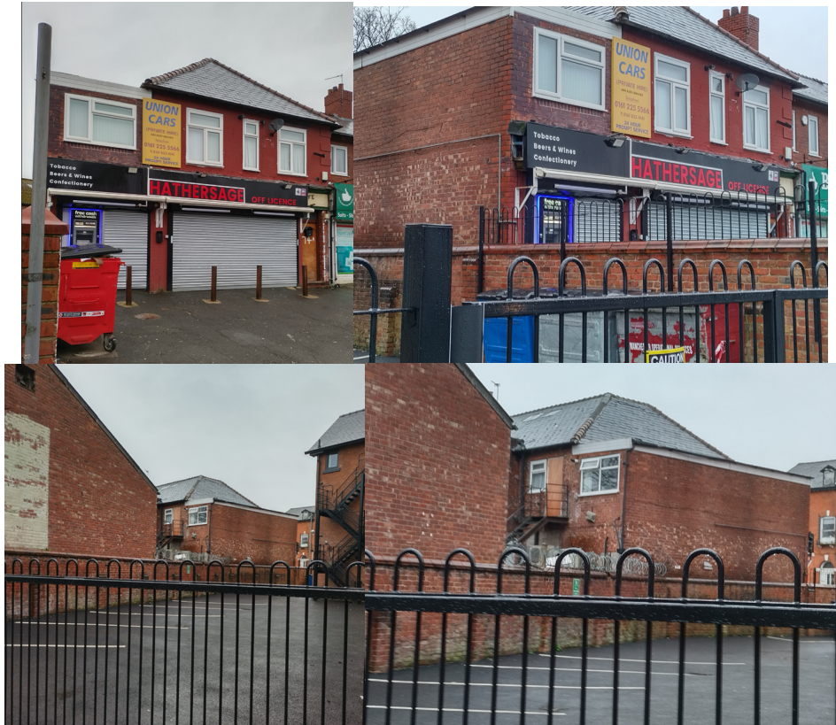
Fig.1 – Views of the application site
