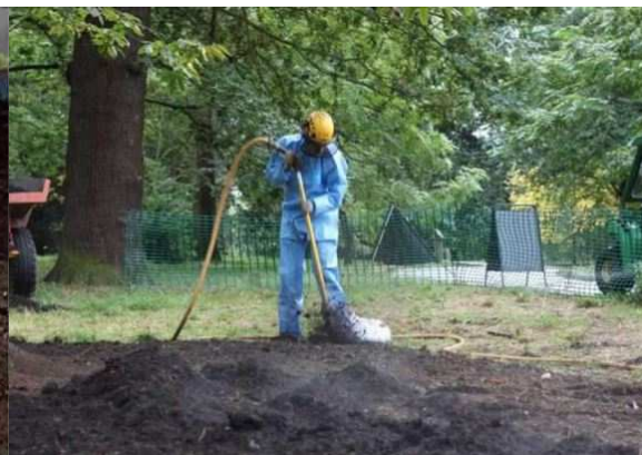
Figure 5: Showing Air-Spade Soil Tilling.
