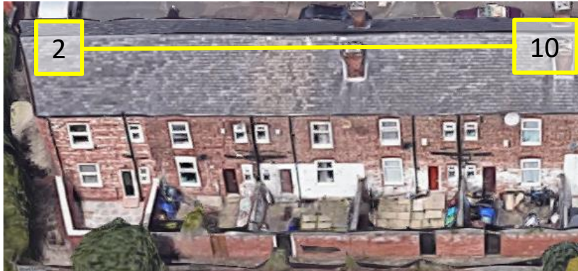
Image 3 - Aerial view of 2-10 Upper West Grove
