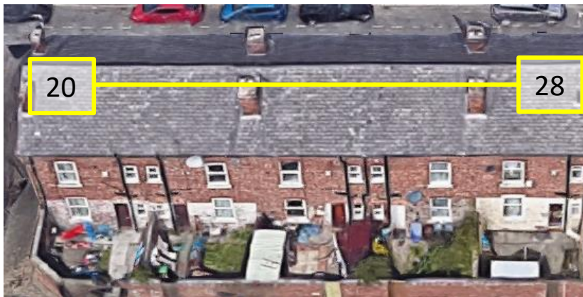
Image 5 - Aerial view of 20-28 Upper West Grove
