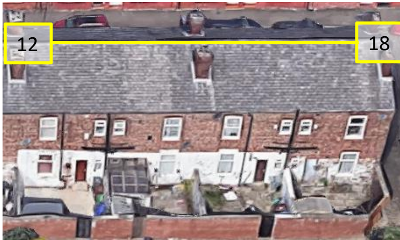
Image 4 - Aerial view of 12-18 Upper West Grove
