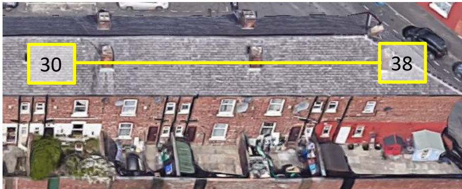
Image 6 - Aerial view of 30-38 Upper West Grove
