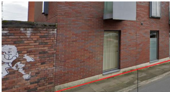
BREWER STREET ELEVATION STONE PLINTH
