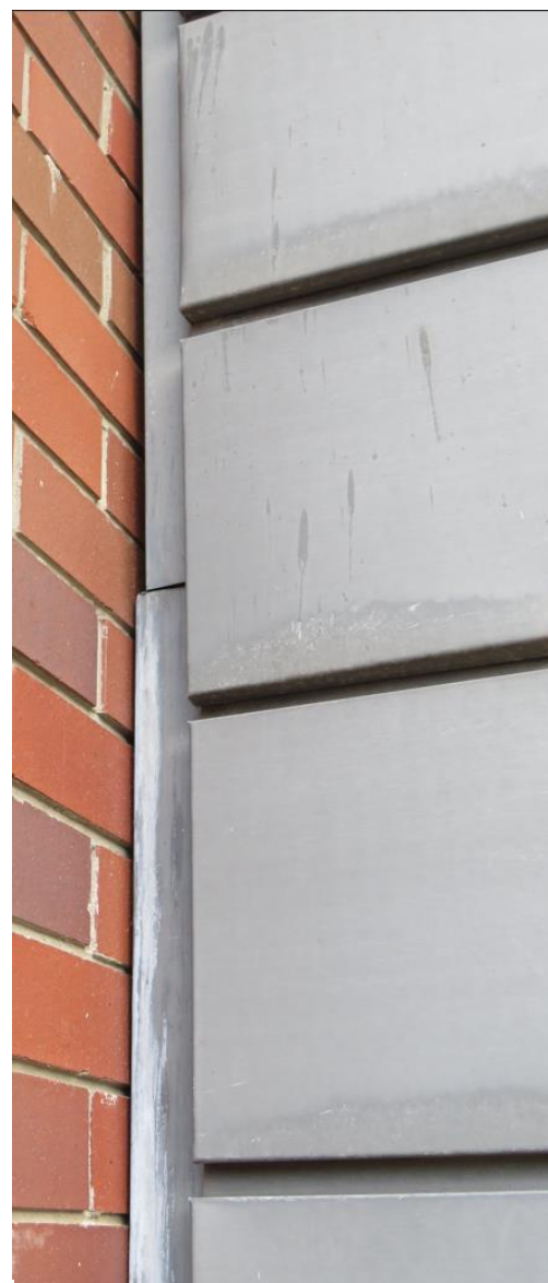
Figure 28 - New zinc panels to replace the glazed panels to match the existing zinc
