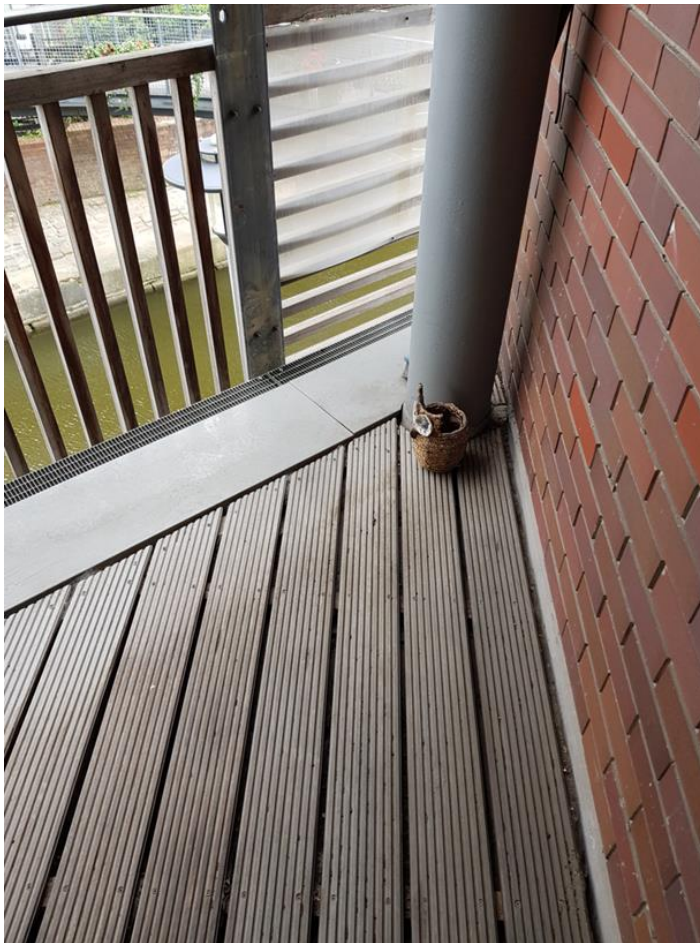
Figure 21 - Existing balcony timber decking
