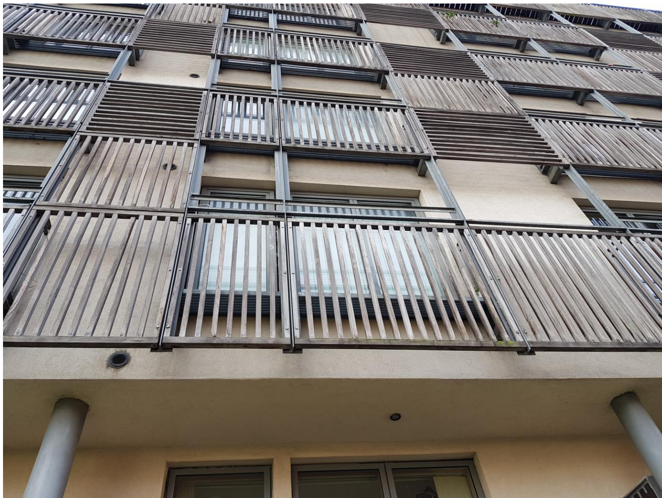
Figure 7 - Detail view of East elevation showing the cream render and timber trellis
