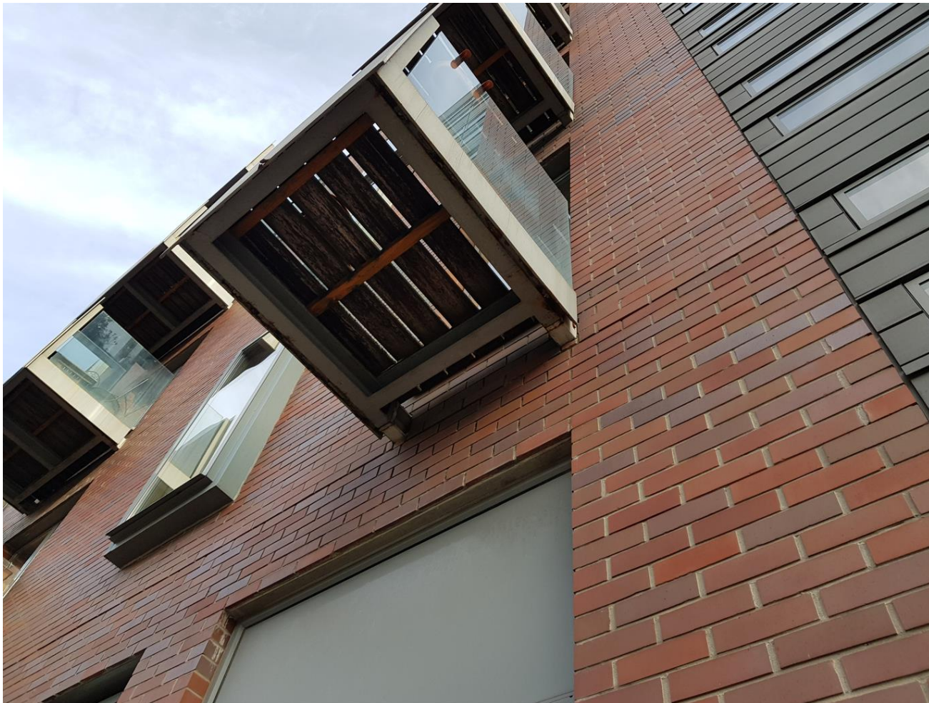
Figure 9 - View of West Elevation showing elevational features / details and brick colours / texture
