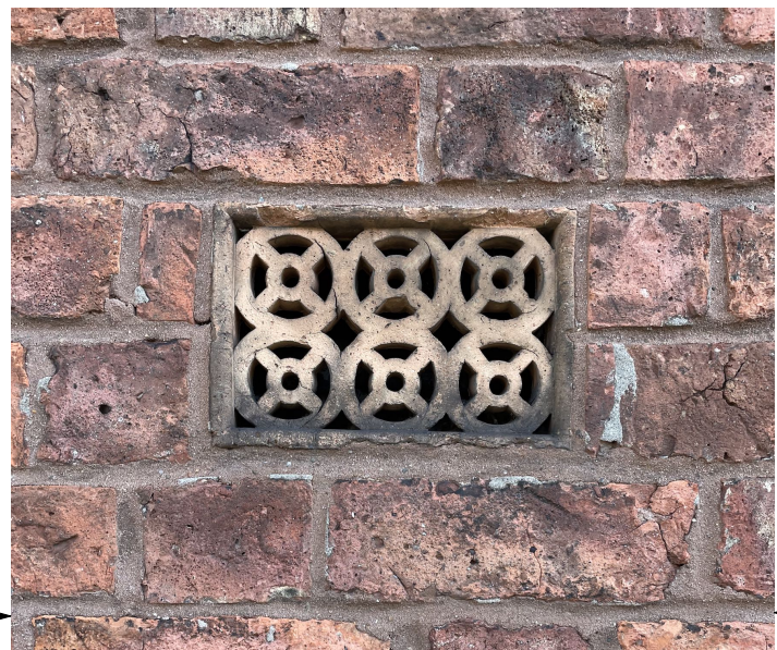
EXISTING 9" x 6" CLAY VENTILATON TERMINAL TO SOUTH & WEST ELEVATIONS
