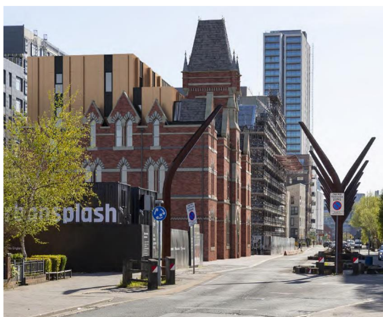
Figure 8.1: View of Ancoats Dispensary looking North East from Old Mill Street (Source: Buttress Architects)
