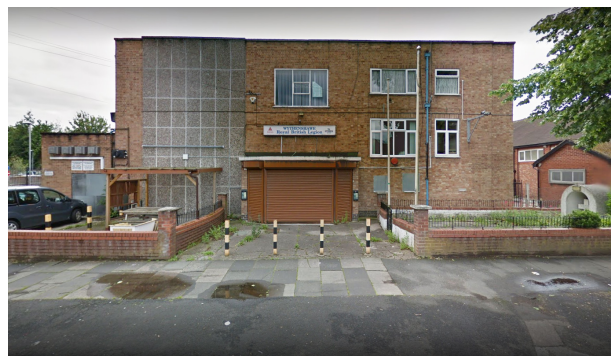
Fig 2. The Royal British Legion, prior to demolition.
